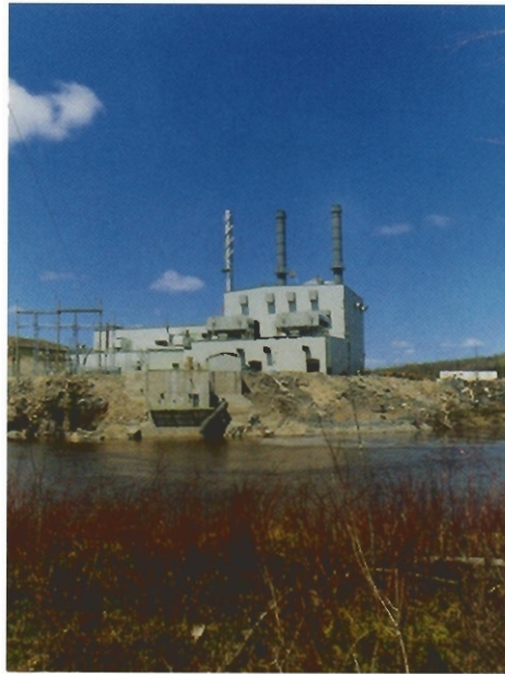
ATCO Noise Management designed, supplied and constructed the acoustic envelope for Northland Power's 104 MW cogeneration plant at Iroquois Falls, Ontario.
