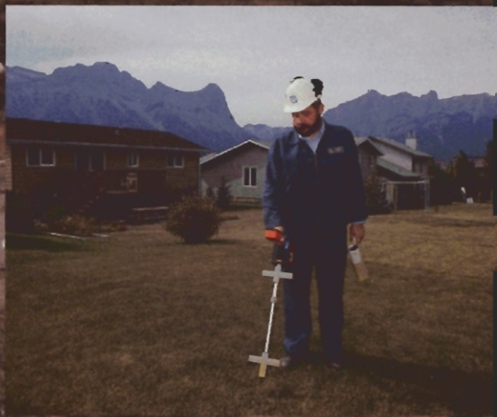
Identifying the location of an underground line.
