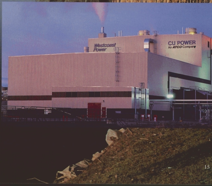
The McMahon Cogeneration plant in Taylor, B.C., provides electricity to the B.C. grid and steam to Westcoast Energy Inc.
