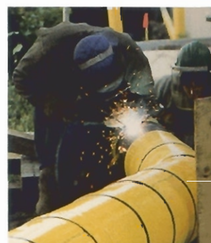
Northwestern Utilities, in the third year of a 10 year, $100 million gas line replacement program, replaced 86 kms of distribution mains and 6,000 services in Edmonton, which were initially installed between 1923 and 1933.
