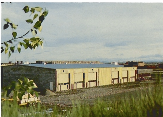
A truck maintenance shop owned by Crone Bros Ltd., Calgary, built of structural steel and cladding manufactured by ATCO Metal.
