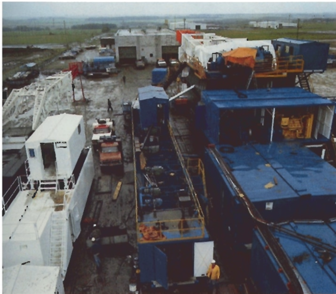
ATCO Drilling's modern maintenance facility at Nisku, Alberta.
