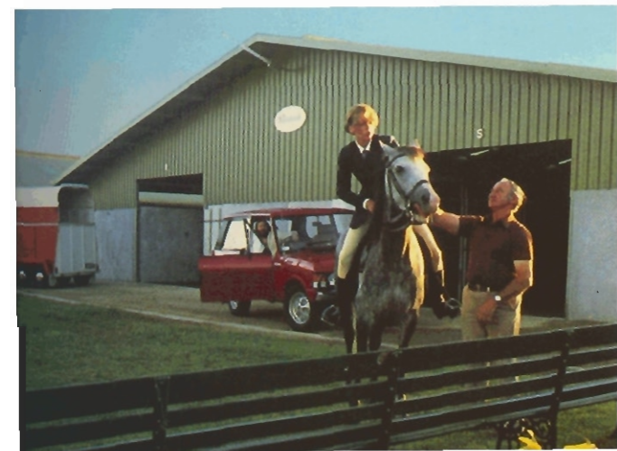
ATCO Supertruss buildings were chosen by the Australian Horse Breeders Co-op Society for their stabling and auction facilities.
