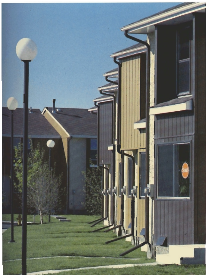
Allenwood, a 57-unit ATCO Housing condominium development in Airdrie, Alberta.
