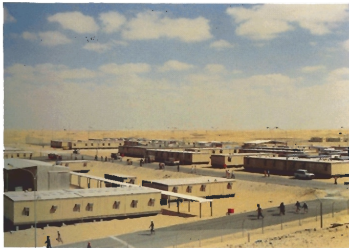
ATCO housing on site for the Abu Dhabi National Oil Company.
