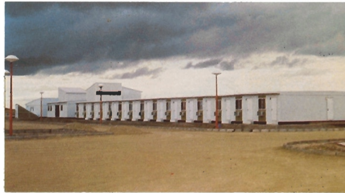
Bottom right: Vessel units under construction for Iraq and Abu Dhabi
