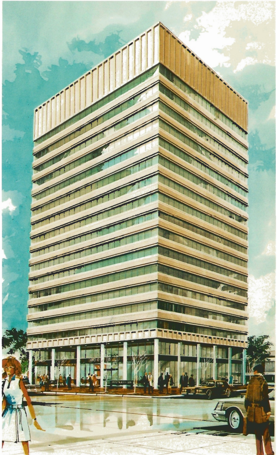
Top left: Construction begins on an 18-storey office complex in downtown Calgary.
