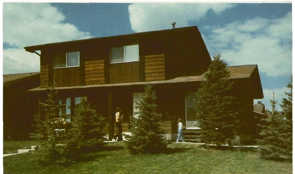
Top: (l-r) R. S. Hegan, General Manager; Rodal, Construction Manager; A. Christ, & J. ... Centre: "Georgian Village", a high quality 234-unit condominium development in Calgary. Right: One of ATCO's affordable but quality housing examples.
