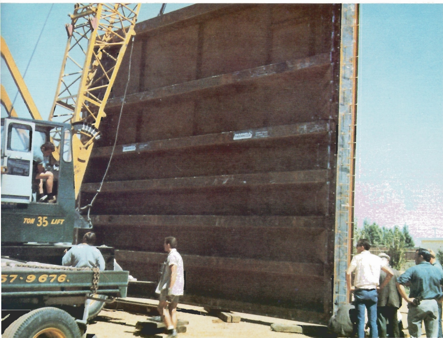
An 18 ton lock gate fabricated by Paraweld for installation on the River Murray irrigation system, in South Australia.
