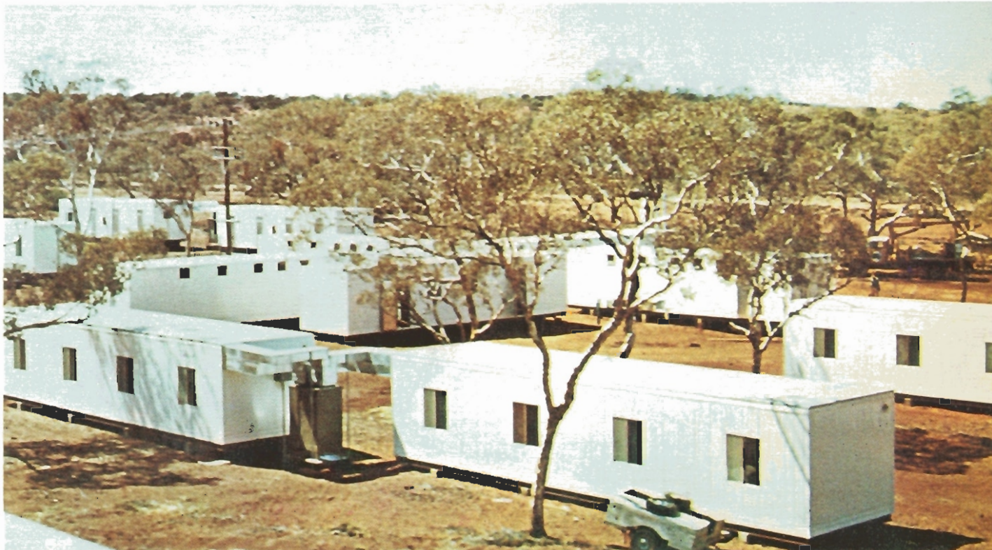
High capacity air-conditioning is featured in this WOWIC housing complex provided for Poseidon to develop their world famous nickel deposits.
