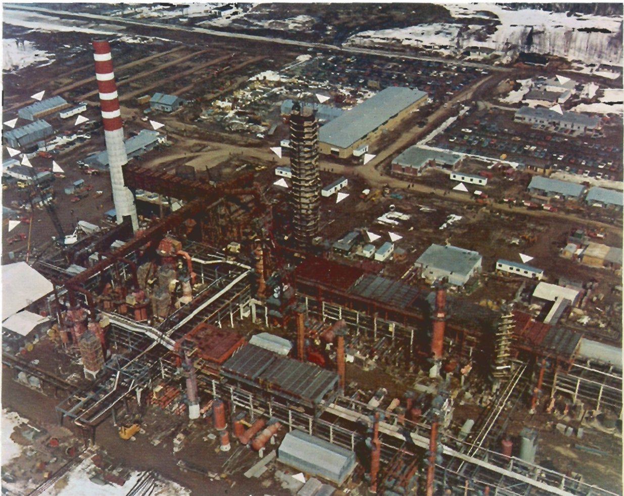
ATCO serves the urban construction market. The Golden Eagle refinery site (pictured here) contains 5 Fold-A-Way buildings and 15 offices.
