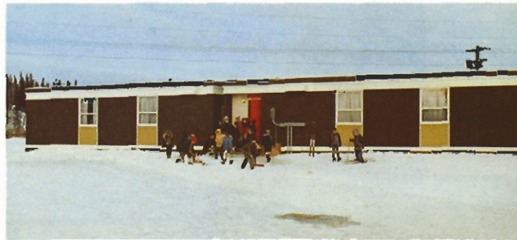
Factory built classrooms continue to be an important product line of ATCO (Western) Ltd. This complex helps to serve the growing population of Fairbanks, Alaska
