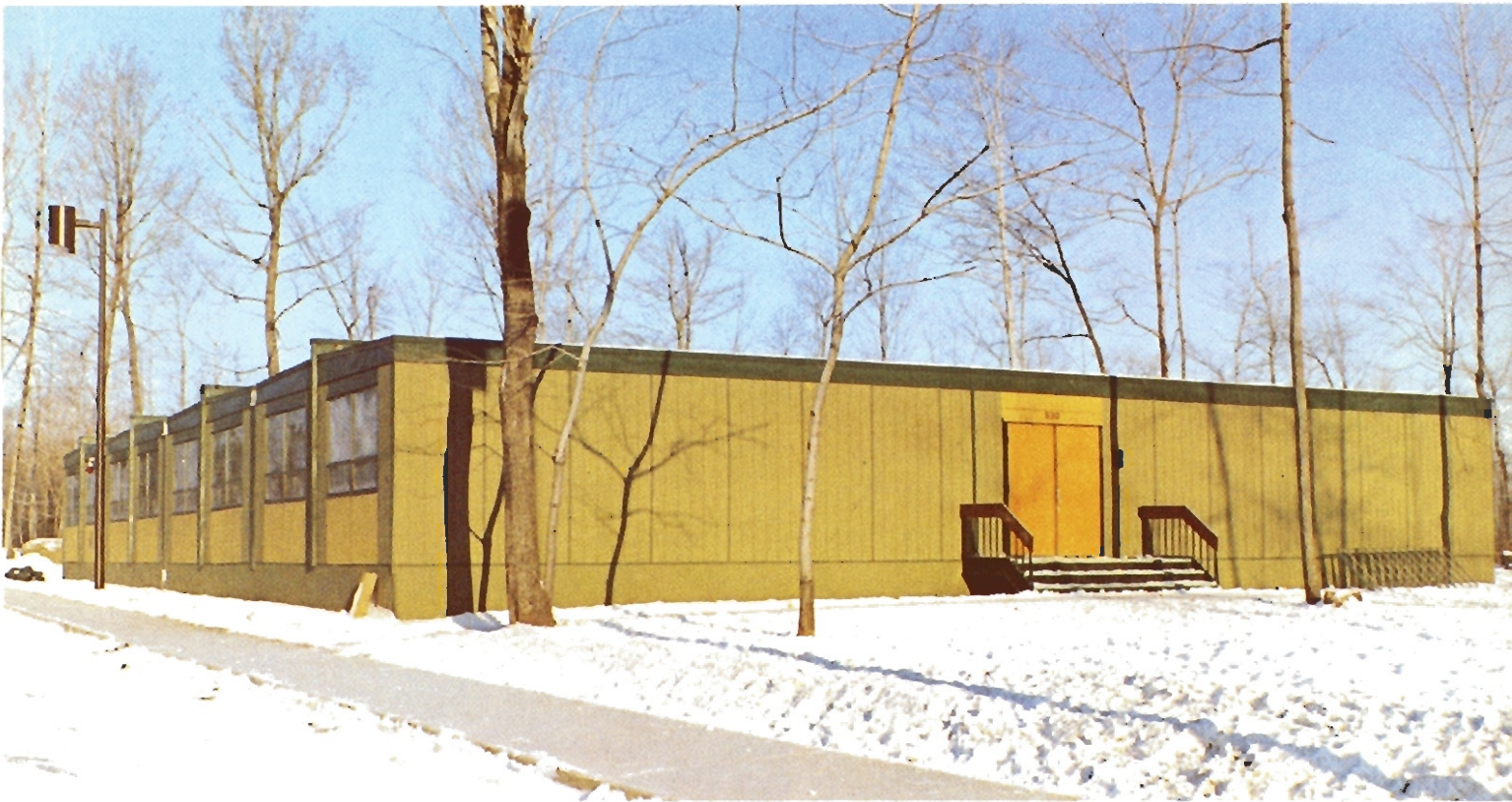
ATCO's relocatable classroom line met continued marketing success during 1969. Although the majority of the classrooms are installed as supplements to existing buildings, there were several instances in which the classrooms were complexed as self-contained, permanent schools. The example illustrated here is an eight-classroom elementary school located on Nun's Island in Montreal.
