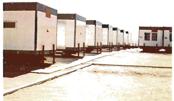
Modern, air conditioned bunkhouses serve a construction camp in the Sahara Desert. These buildings were constructed for an Italian company operating in Algeria. At right is a portion of a large kitchen dining complex.
