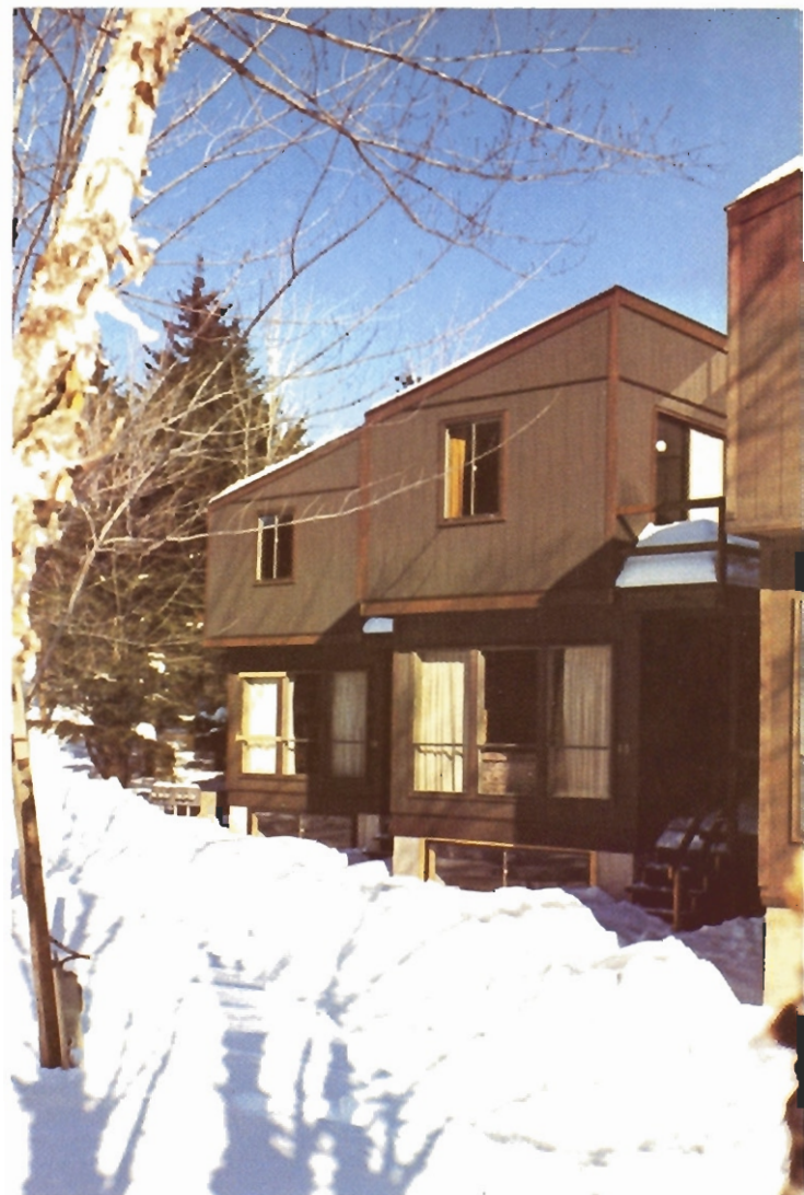
This unique ski lodge in Vermont was built of factory constructed, transportable modules, which were stacked two deep upon delivery. The experience ATCO has gained in building industrial structures is leading the company into the manufacture of many types of community structures.
