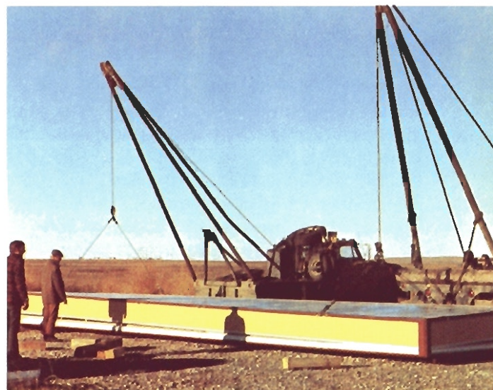
Under the Program for the Advancement of Industrial Technology (P.A.I.T.) sponsored by the Canadian government, the R & D Centre has designed an improved building system for export structures. The building appears above in its shipping configuration, below, in its deployed form.
