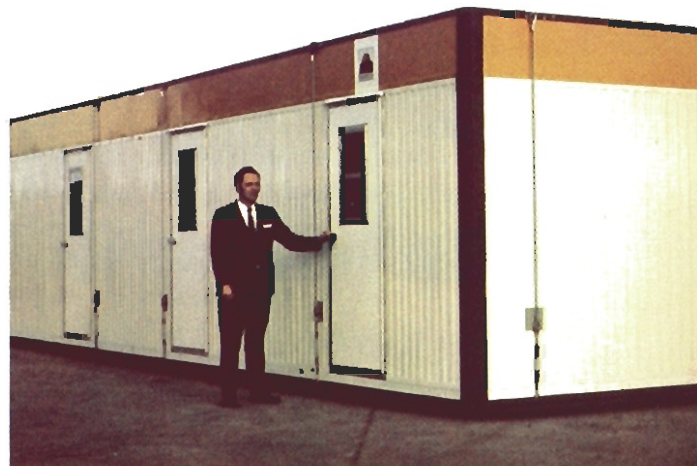
The R and D Center's Airmobile Maintenance Shop (A.M.S.) offers a vertical expansion of 2:1. The building is constructed of a unique honeycomb, sandwich panel material developed by the company.
