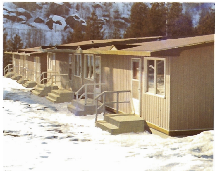
This senior citizens' home was installed at Castlegar, British Columbia, early in 1969. Comfortable and aesthetically pleasing, the building illustrates the urban potential for systems built structures.
