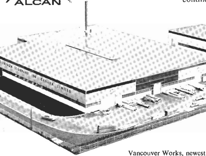
Vancouver Works, newest fabricating plant of Aluminum Company of Canada, Limited, produces rod, cable and extrusions
