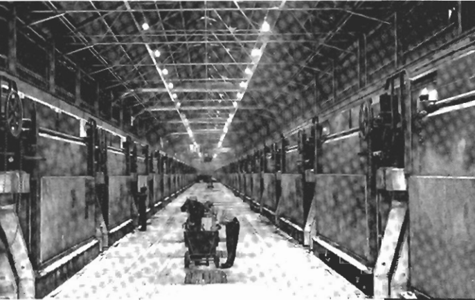
Interior view of Isle Maligne, Quebec smelter showing two rows of smelting pots
