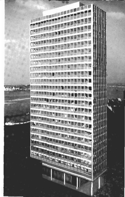
Headquarters of two West German steel companies in Dusseldorf use aluminum window and wall systems.
