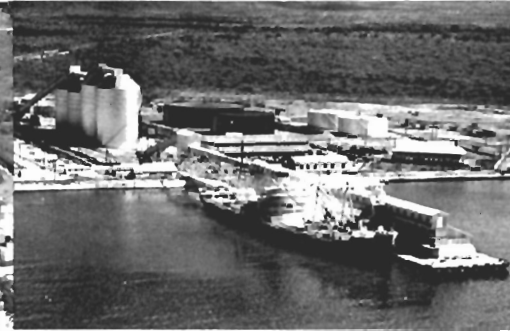
Port Esquivel, built on the south coast of Jamaica by the Company, discharges 1,000 tons of alumina per hour into the ships' holds
