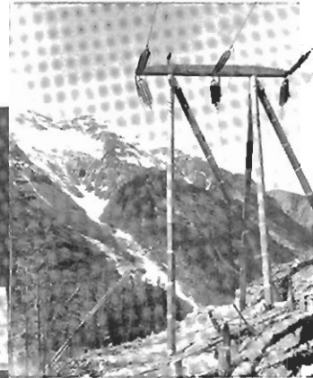
Aluminum towers carry one set of transmission lines over Kildala Pass from Kemano to the Kitimat smelter
