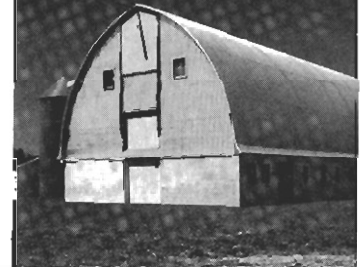
Aluminum barns have low annual cost, and being cooler, improve animal yields
