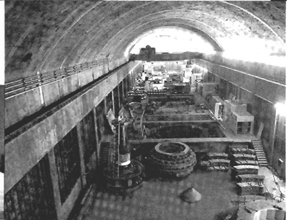
The Chute-des-Passes underground powerhouse has five generators with a total capacity of 1 million h.p. Three generators went on power in 1959
