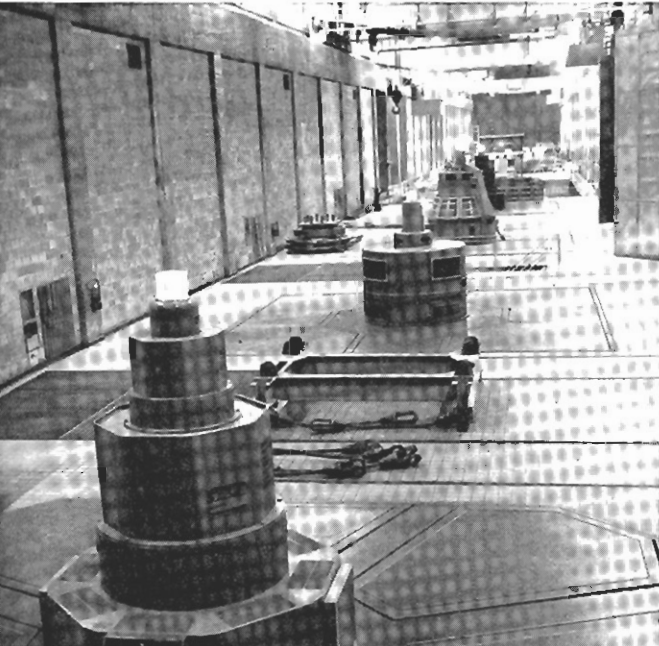
Kemano powerhouse has seven generators in operation with a capacity of 1,050,000 h.p. This supplies Kitimat smelter
