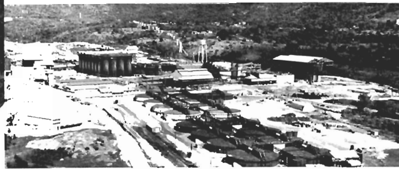
Alumina Jamaica Limited's new ore refining plant at Ewarton has a capacity of 270,000 tons of alumina per year
