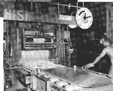
South Africa. Hot rolling sheet in the Pietermaritzburg plant of Aluminium Company of South Africa (Pty.) Limited
