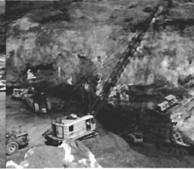
Open-pit mining of bauxite in Jamaica. The ore is transported by carry-all vehicles to the Kirkvine plant
