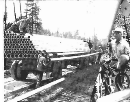
Aluminum pipe for water injection, Pembina oilfield, Alta. Inset: Alcan portable pipe welder in use
