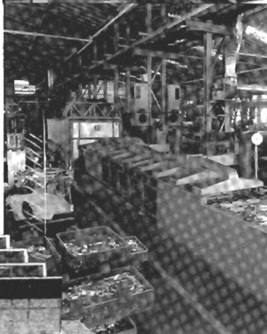
Germany. Slugs for containers emerging from the annealing furnace on the conveyor in the plant of Aluminiumwerke Göttingen G.m.b.H.
