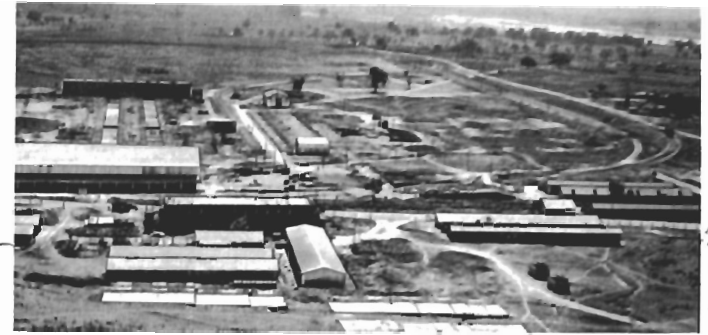
INDIA The new 11,000 ton per year smelter of the Indian Aluminium Company, under construction near Hirakud, Orissa, to be powered by state hydro project.
