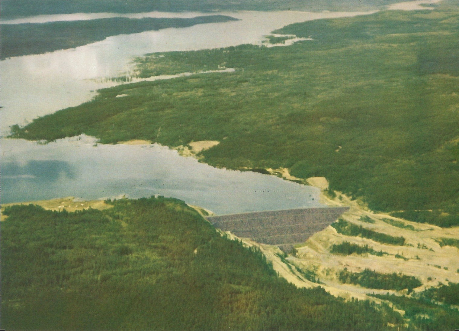
Kenney Dam at the east end of the 350 square-mile reservoir, tapped at the west end by a ten-mile tunnel which drops the water half a mile to the Kemano turbines.
