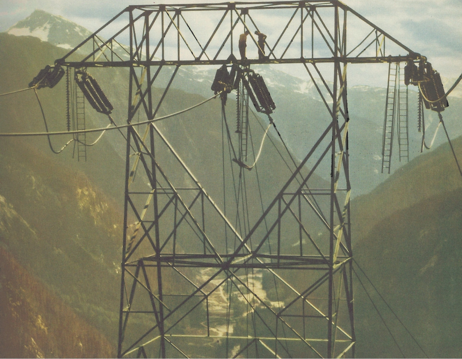
Aluminum conductor cables being strung on a steel transmission tower high above the Kemano River valley.
