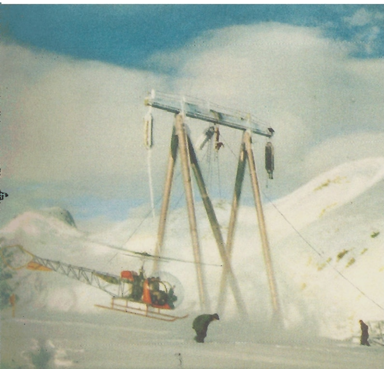
Aluminum conductor cables being strung on a steel transmission tower high above the Kemano River valley.
