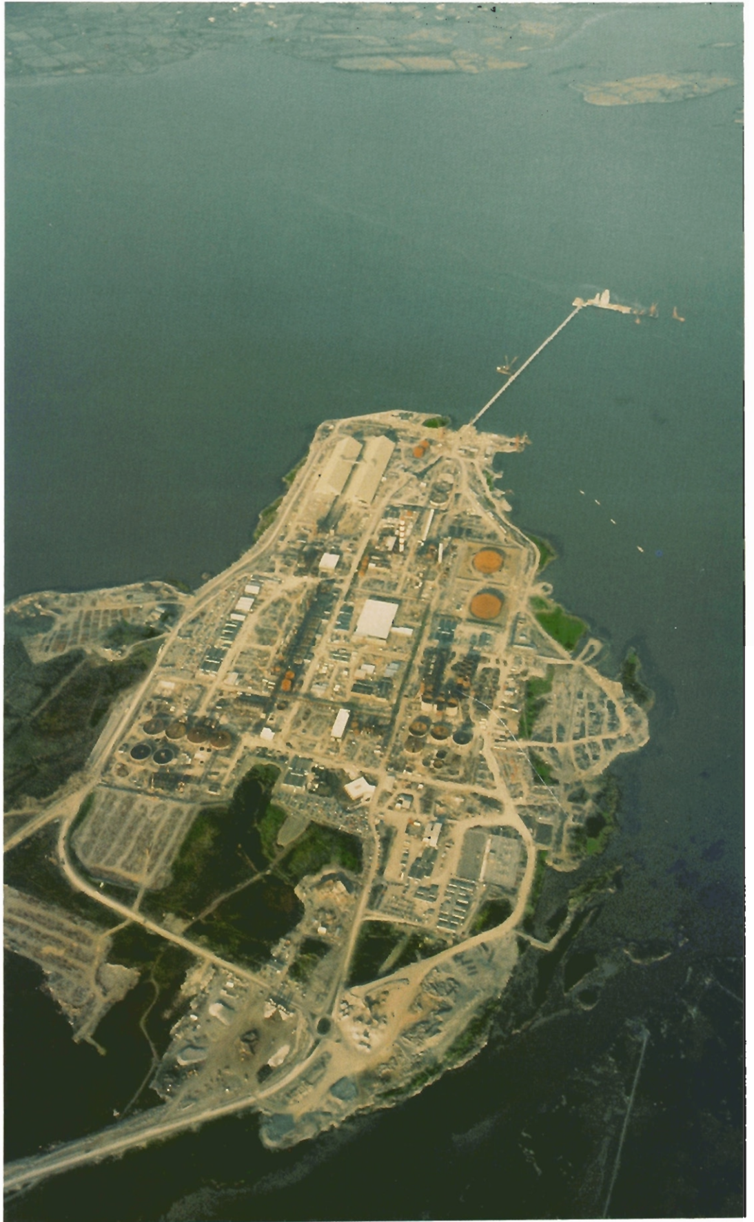
Aughinish alumina plant on the Shannon River in Ireland, will have an annual capacity of 800,000 tonnes when completed in 1983.
