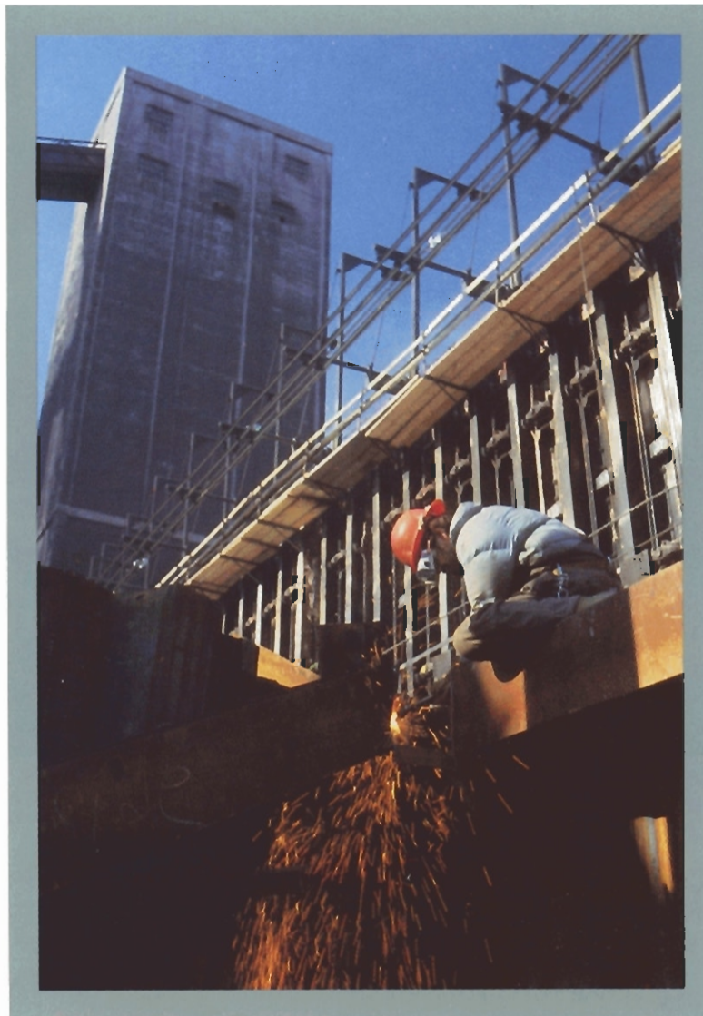
No. 8 coke oven battery modifications underway.
