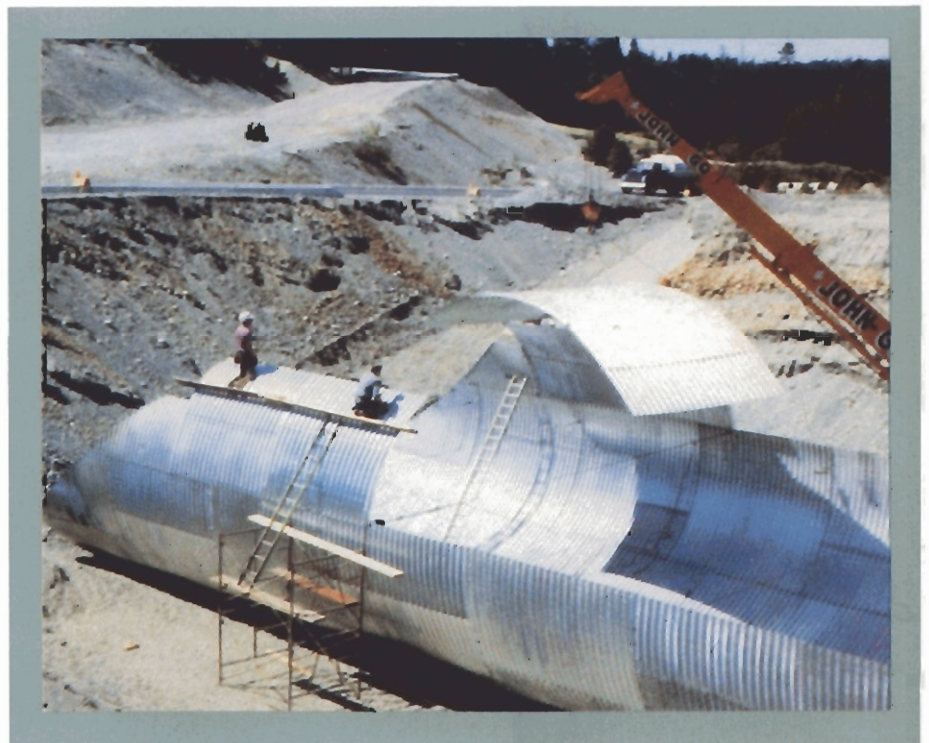
Algoma's hot rolled sheet, up to 8 feet wide, is used in these large corrugated highway structures.
