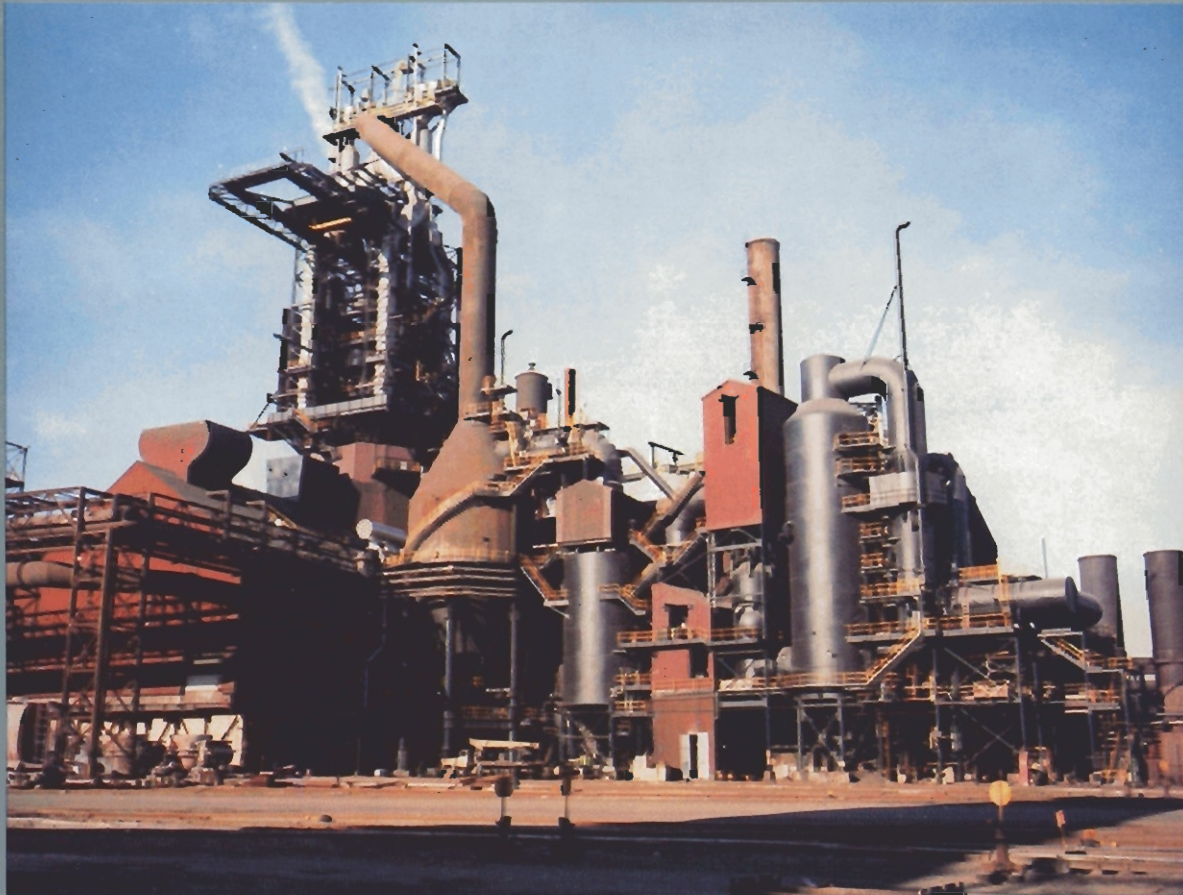
No. 7 blast furnace was relined and modernized in 1981.
