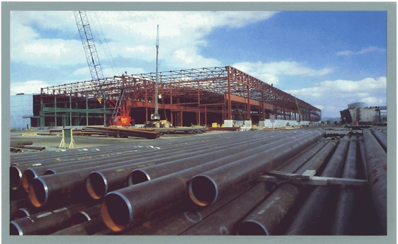
New seamless tube mill under construction.
