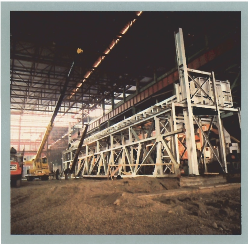
Reheat furnace under construction in the new seamless tube mill.
