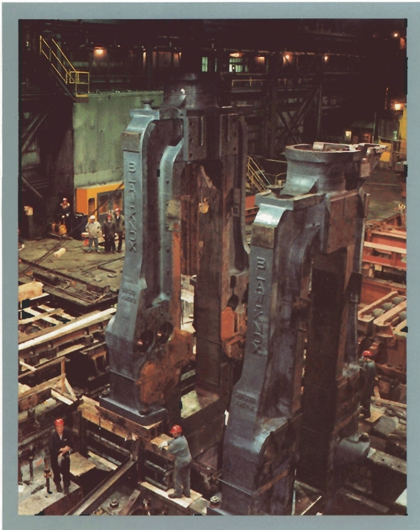
46" slabbing mill housings replaced during mill rehabilitation program.
