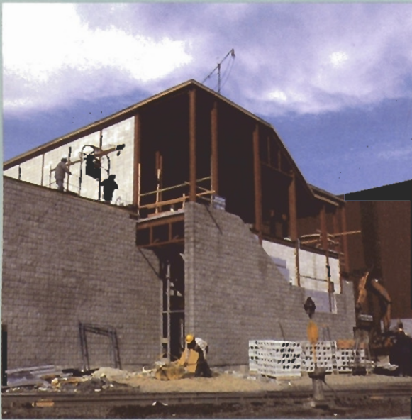
Modern welfare facility under construction to accommodate Algoma employees.
