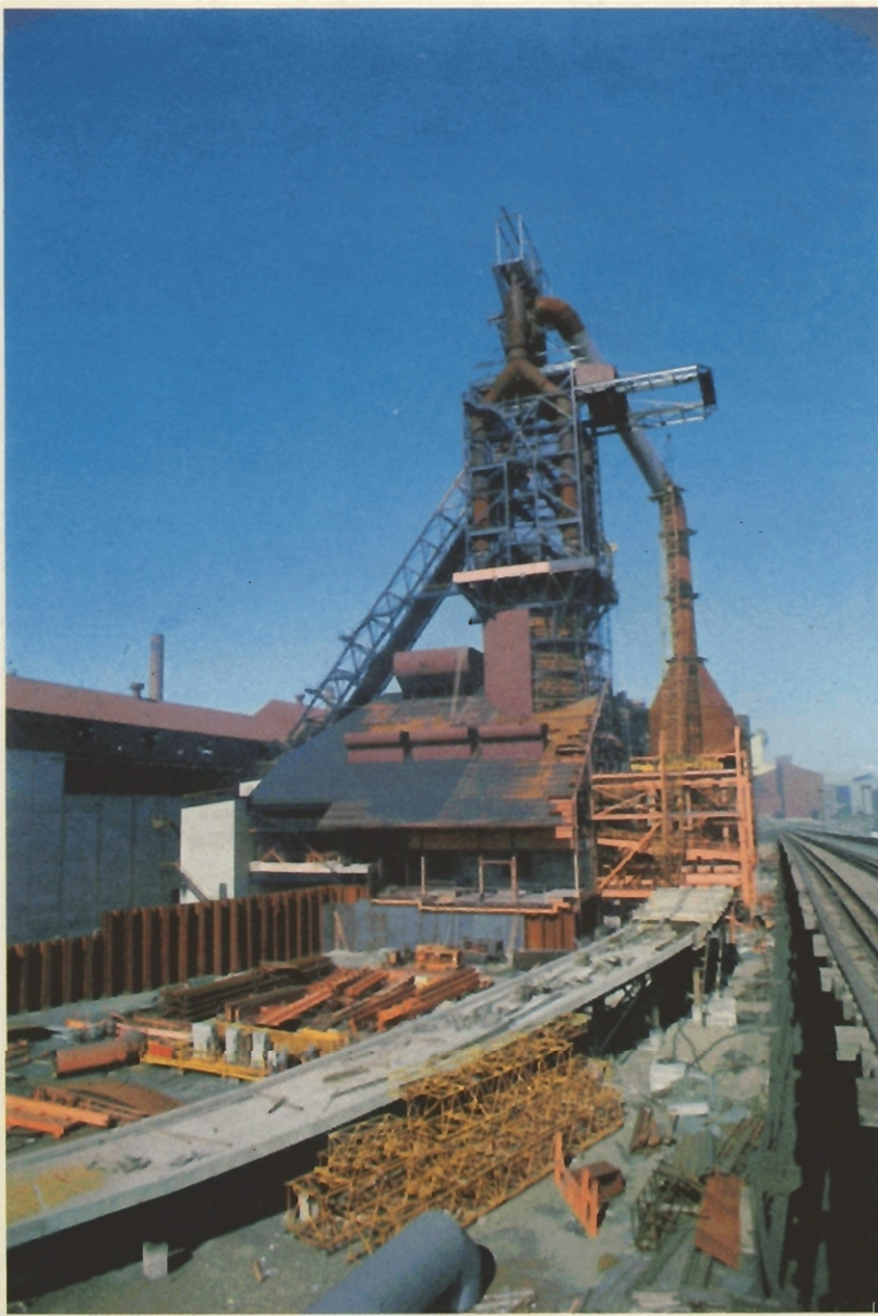
Top—No. 7 blast furnace will increase total hot metal availability.
