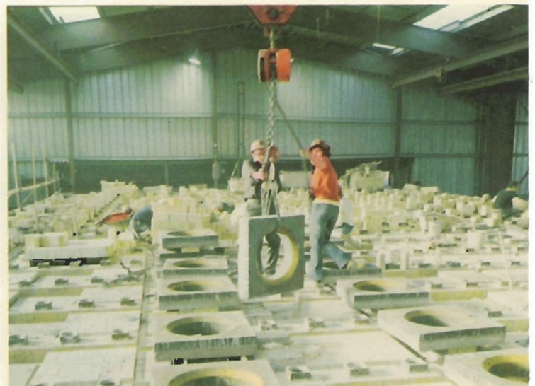
Bottom Right—Locating refractory shapes on the top of No. 9 coke oven battery.
