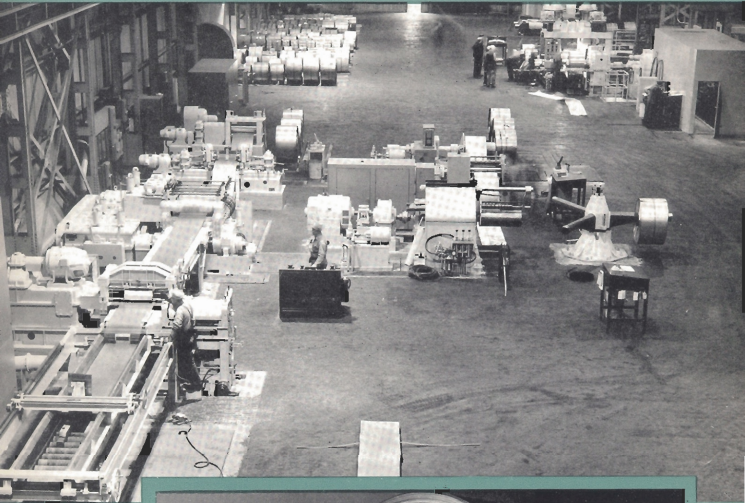
Cold Strip Shearing Operation
