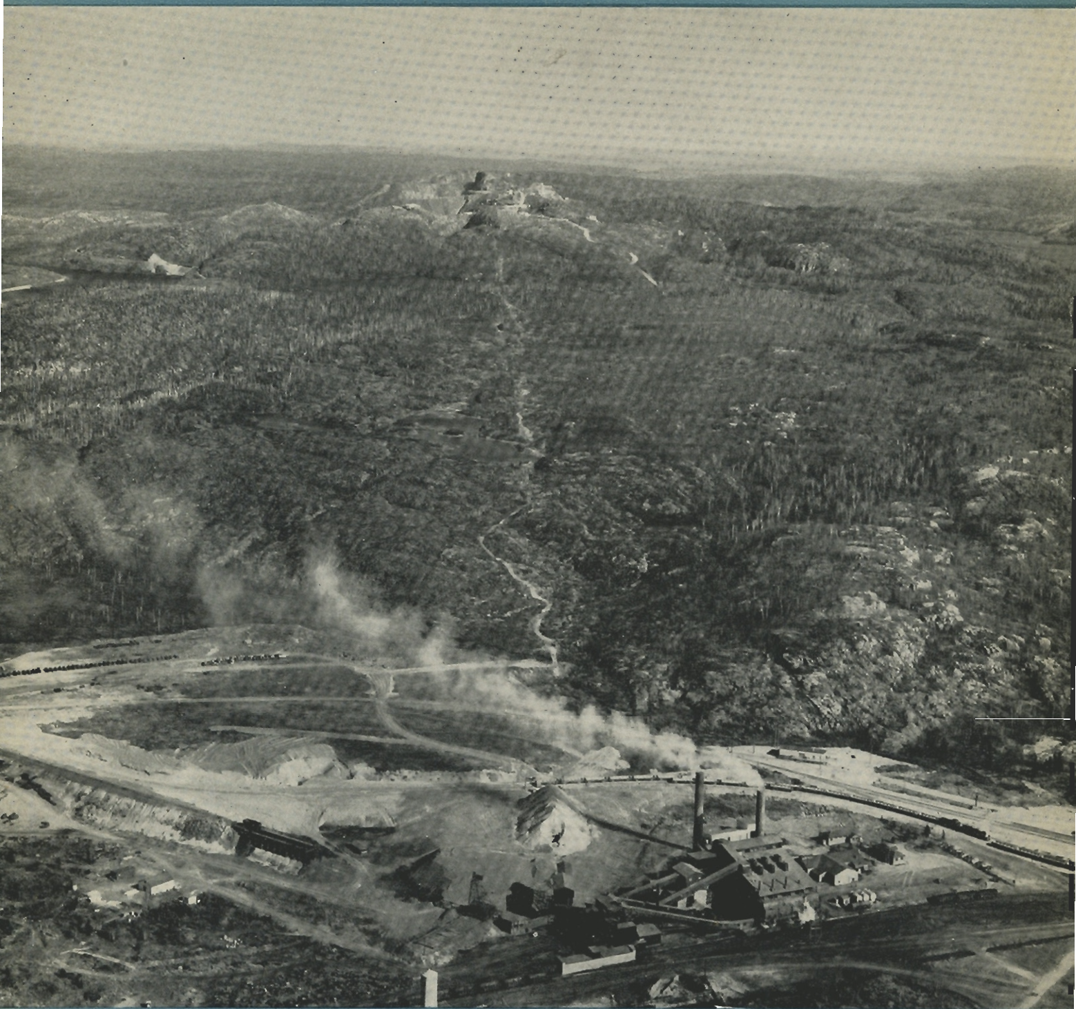
Algoma Ore Properties Sintering Plant with Helen Mine in background
