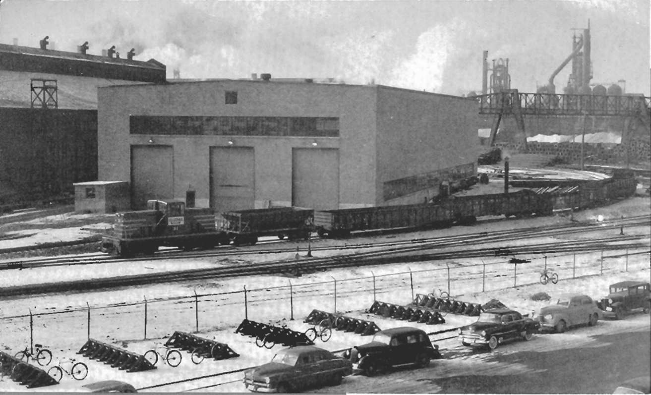
New Diesel Electric Maintenance Building for servicing thirteen new diesel electric locomotives
