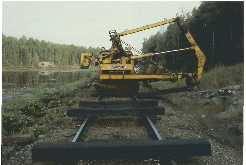
Replacing railway ties.
