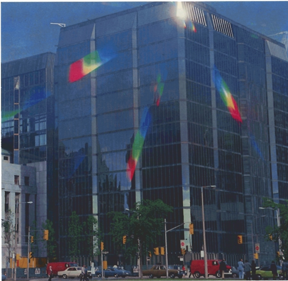
From top left, clockwise: Bank of Canada building, Ottawa, uses aluminum extrusions to frame its 20,000 m 2 of curtain wall.
