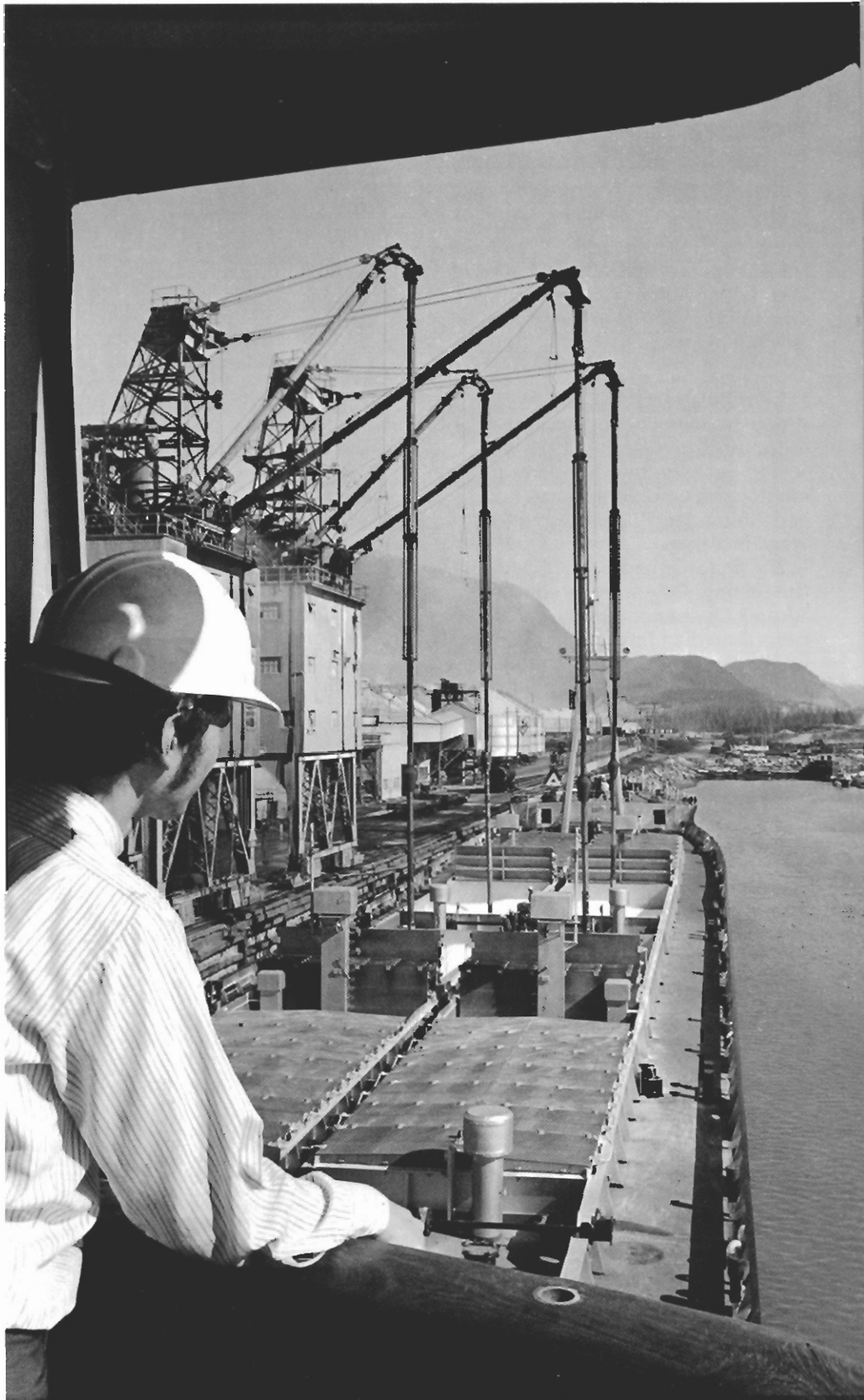
At Kitimat harbour, British Columbia, suction-type unloaders draw, from the hold of an ocean-going ship, the powdery
