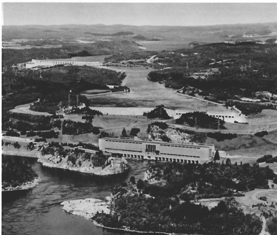
Two of Alcan's six hydroelectric plants in the Saguenay-Lake St. John region system. Upper left: Chute-à-Caron, with an installed capacity of 224,000 kilowatts, was
