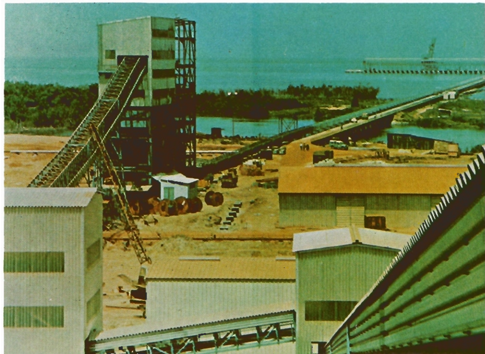
Boké Project in Guinea, West Africa. The newly-completed Port Kamsar where bauxite is crushed, dried and
