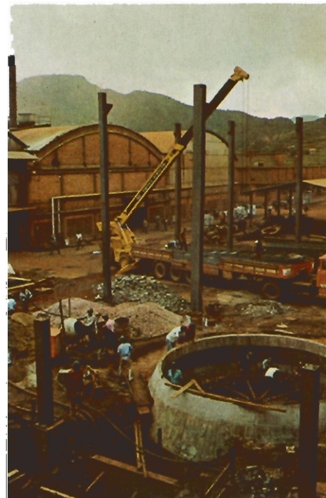
Additional furnaces are installed for the production of ferro-alloys at the Saramenha complex, Brazil.
