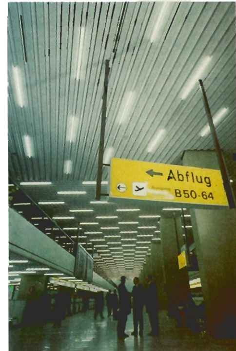
Pre-painted, perforated aluminum sheet cuts down noise, enhances appearance at the new Dusseldorf airport terminal.
