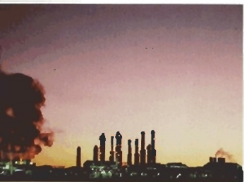
Cold winter air and a dazzling sunset combine to bathe the Cochrane plant in a portrait of rose colored light and rising steam.
