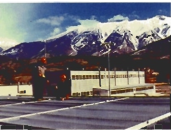
The Croisneest Compressor Station No. 1 was constructed in 1960 and 1961 as part of the 1,700 mile Alberta-California natural gas pipeline system.
