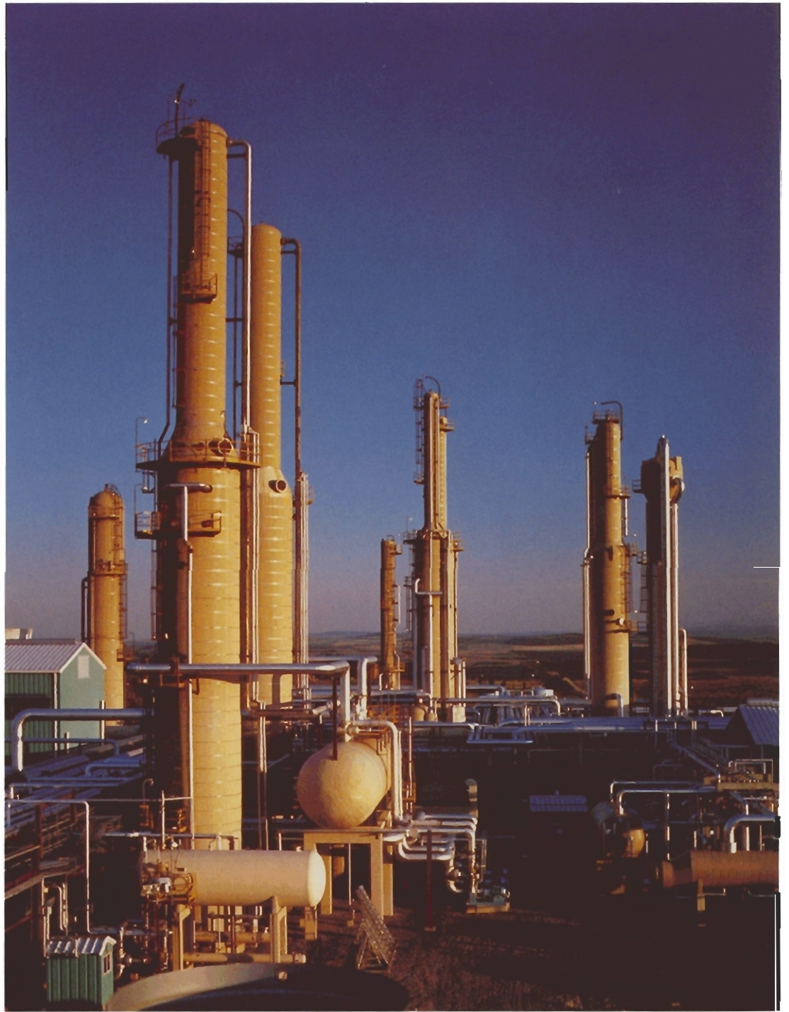
Alberta Natural Liquids Extractor Plant, as seen from the North
