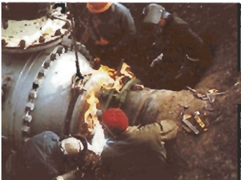
A giant valve is installed on the Alberta-California natural gas pipeline project in 1962.
