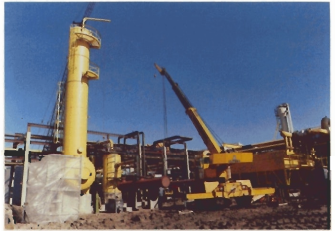
Installation of new CO 2 removal unit.
