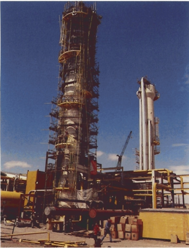
Insulating new demethanizer tower at Cochrane.
