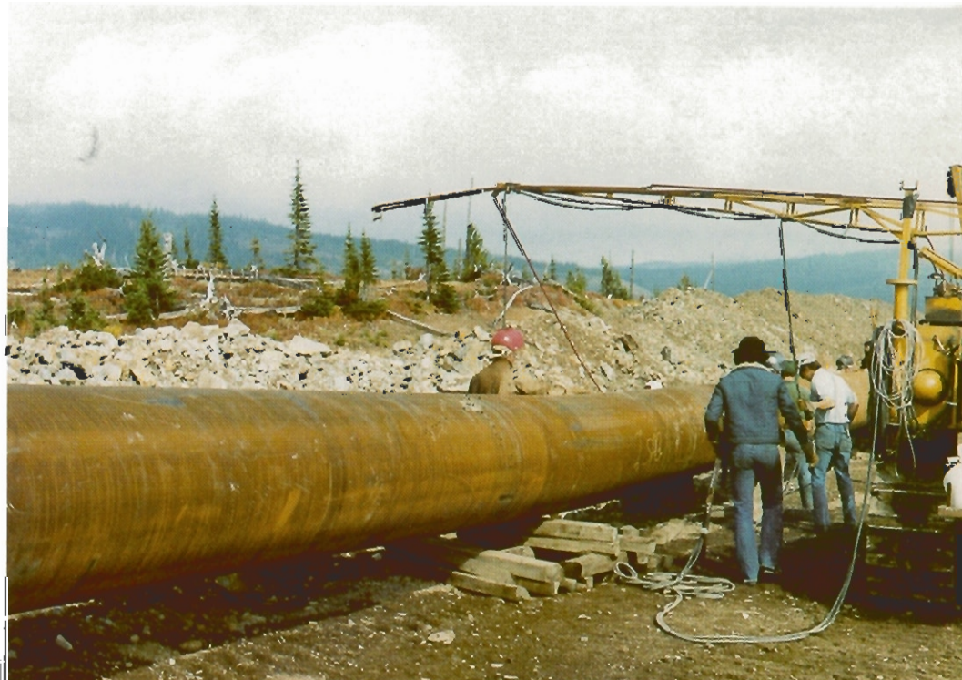
View of welding operations near the top of Flathead Ridge.
