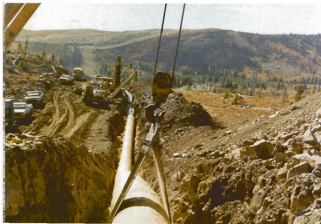
View of lowering-in a section of new pipeline on Flathead Ridge.
