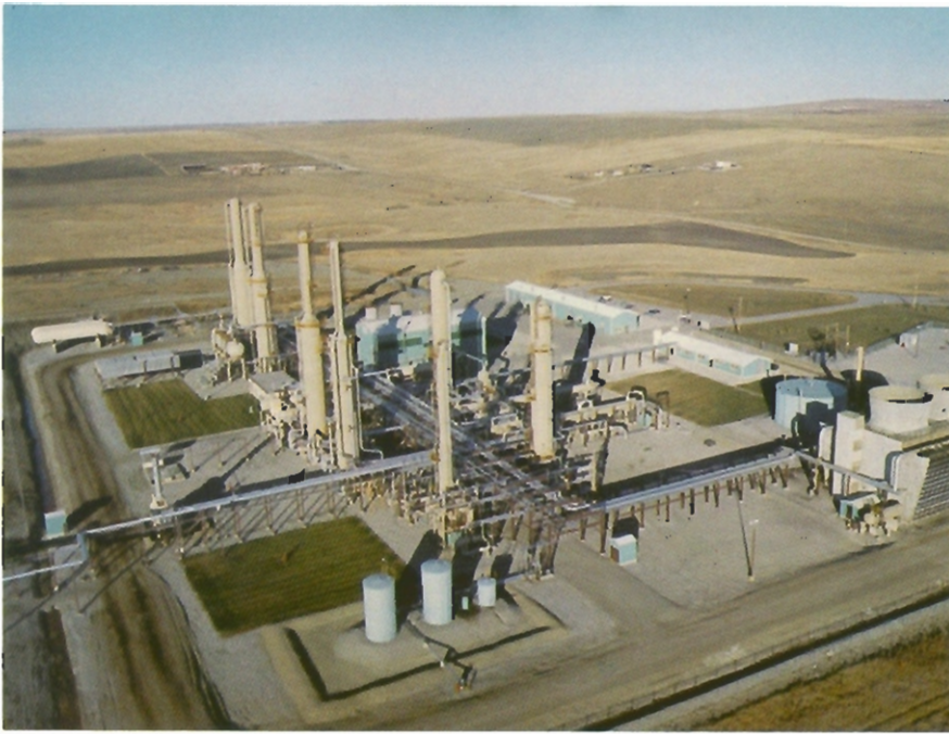
Aerial view of Alberta Natural's Cochrane liquids extraction plant.
