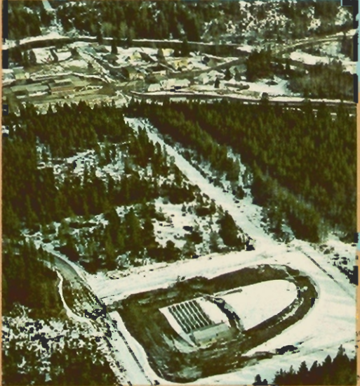
Kingsgate Meter Station at the international boundary
