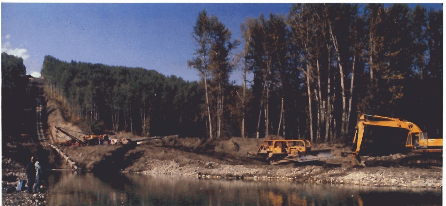
Wapiti River Crossing, 406.4 mm (16-inch) pipeline construction near Elmworth, Alberta
