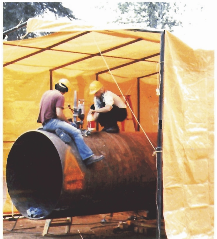
Welding test pipe, Rainbow Lake burst test facility, Alberta
