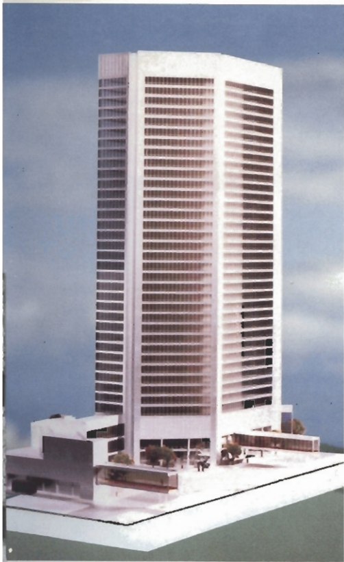
AGTL head office building (under construction)
