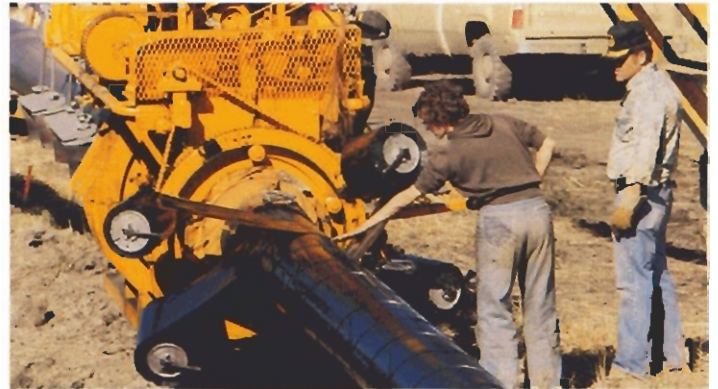
Coat and wrap, 406.4 mm (16-inch) pipeline construction near Elmworth, Alberta
