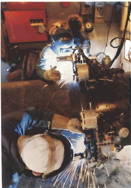
Automatic welding, 762 mm (30 inches) pipeline construction near Peace River.
