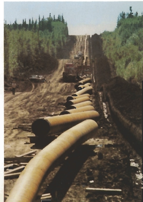
762 mm (30 inches) pipeline construction near Peace River.
