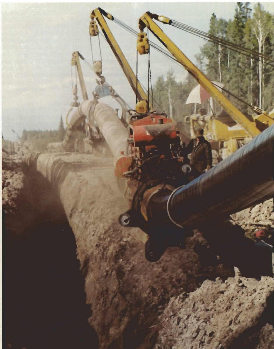
Coat and wrap, 762 mm (30 inches) pipeline construction near Peace River.
