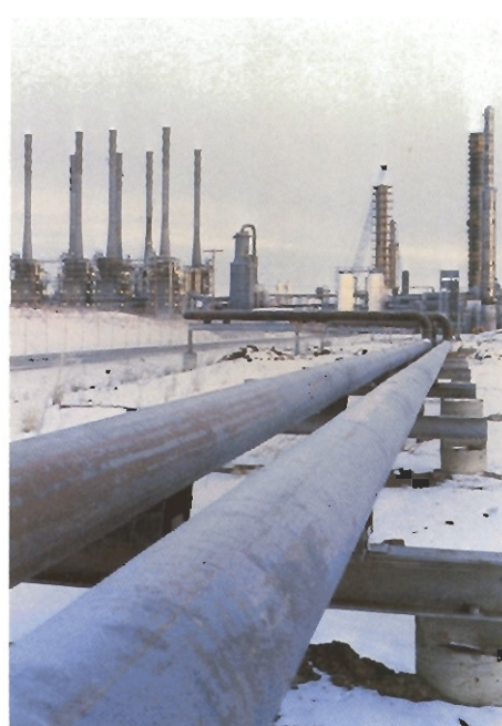
AGECL ethylene plant under construction, Joffre, Alberta.
