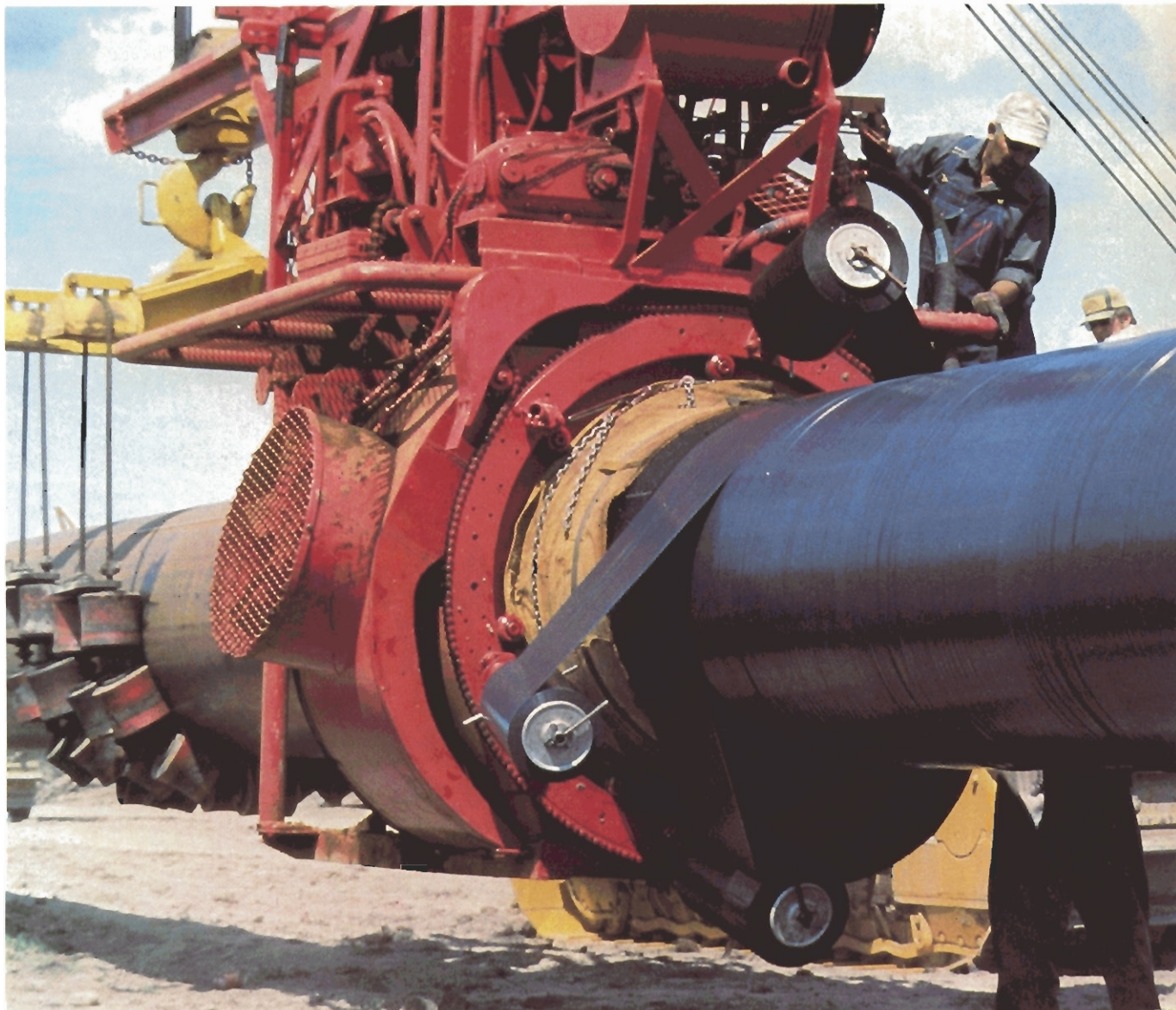
Coating and wrapping pipe on a 42-inch project.
