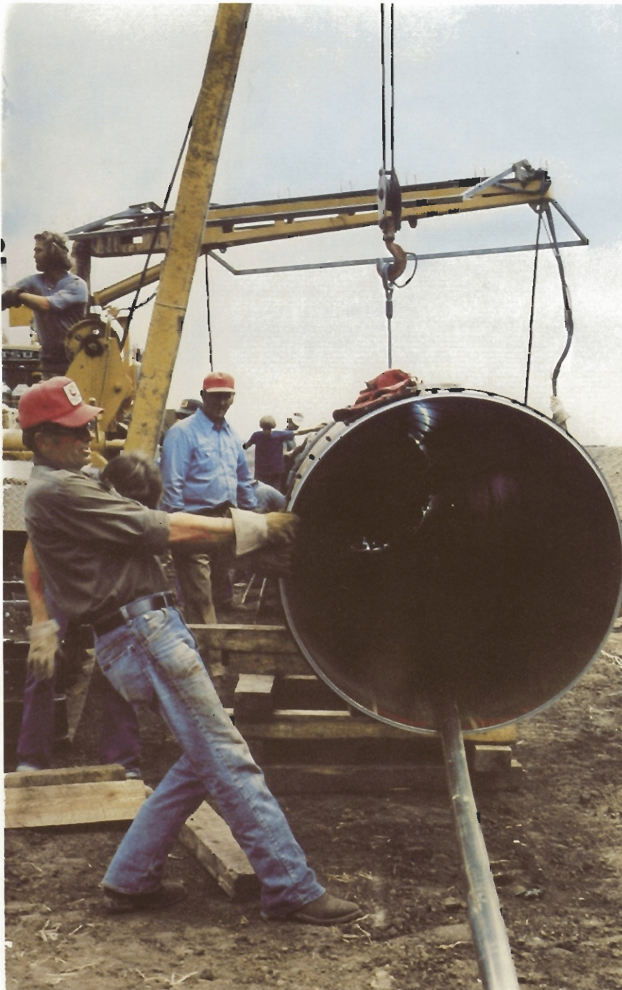
Internal automatic welding on the 42-inch Carstairs project.
