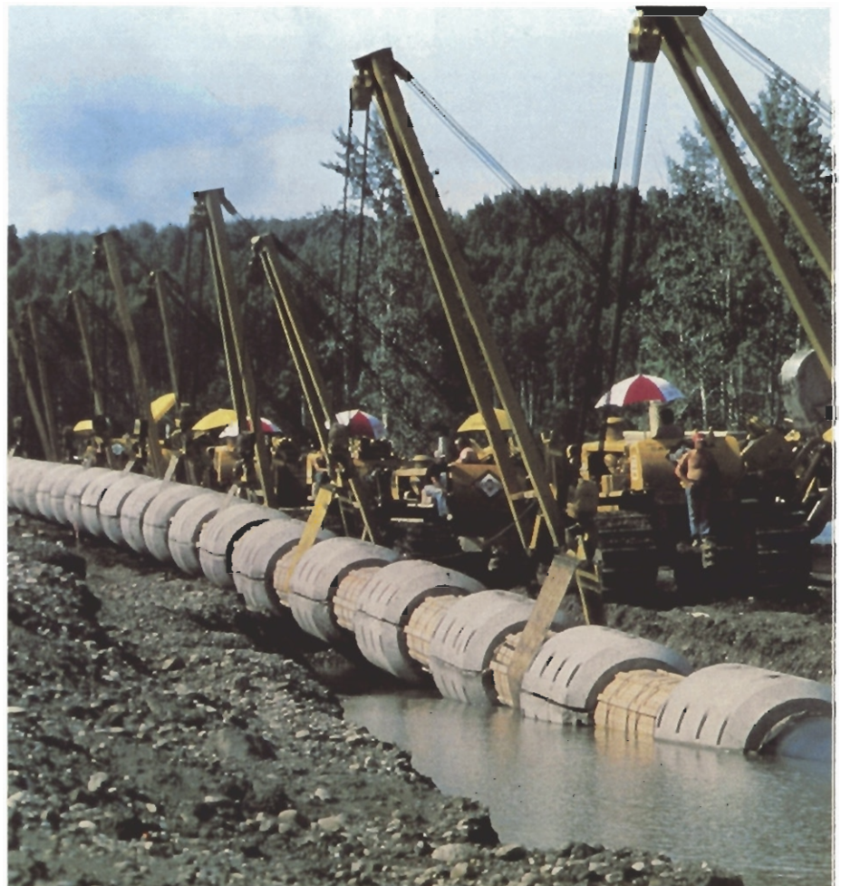
Pipeline river crossing.
