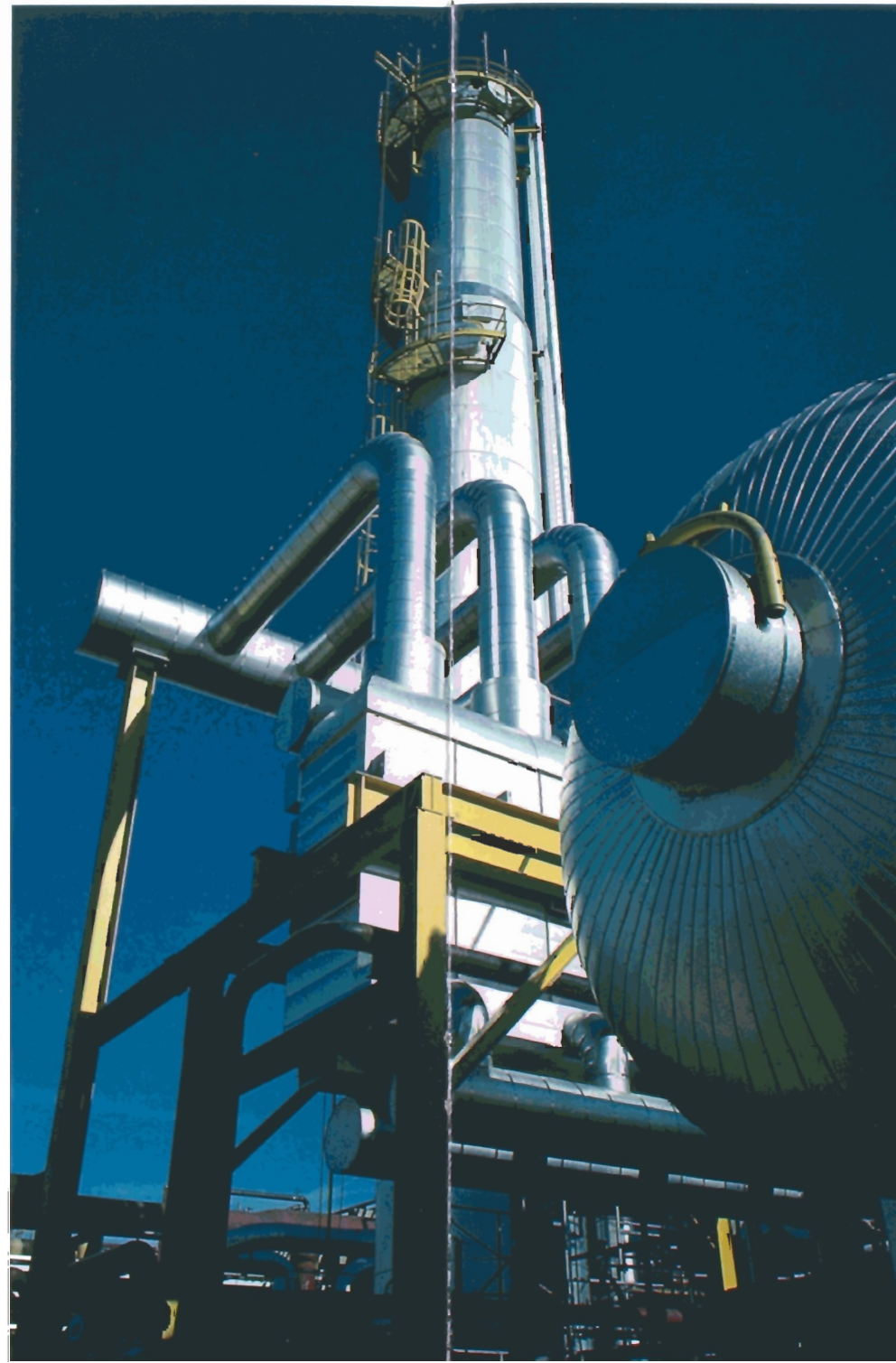
The natural gas liquids extraction plant strips out the heavier components - ethane, butane, propane - from the gas stream prior to the gas being shipped out of Alberta.
