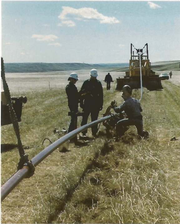
Construction of gas gathering system
