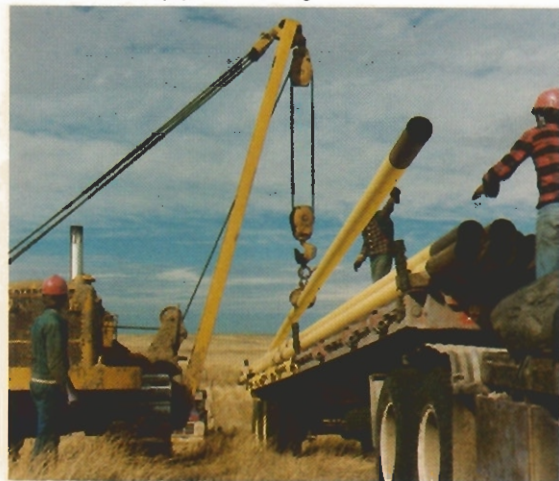
Below: Suffield pipe unloading
