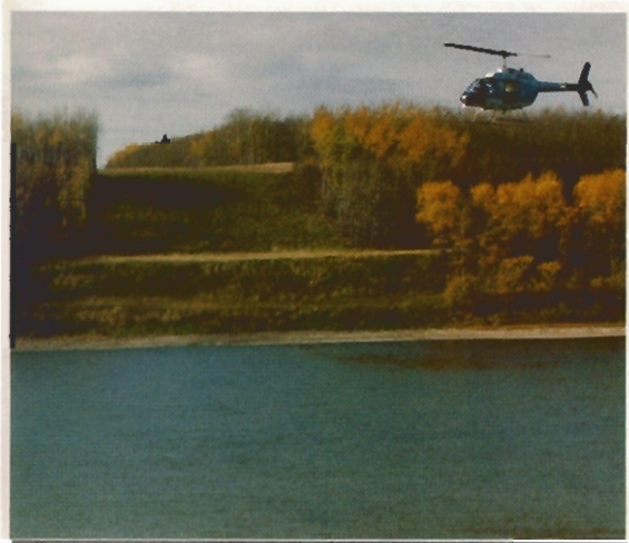
Above: Helicopter patrol, remote control centre and pipeline alley.
