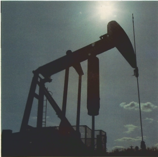
Oil well pumper
