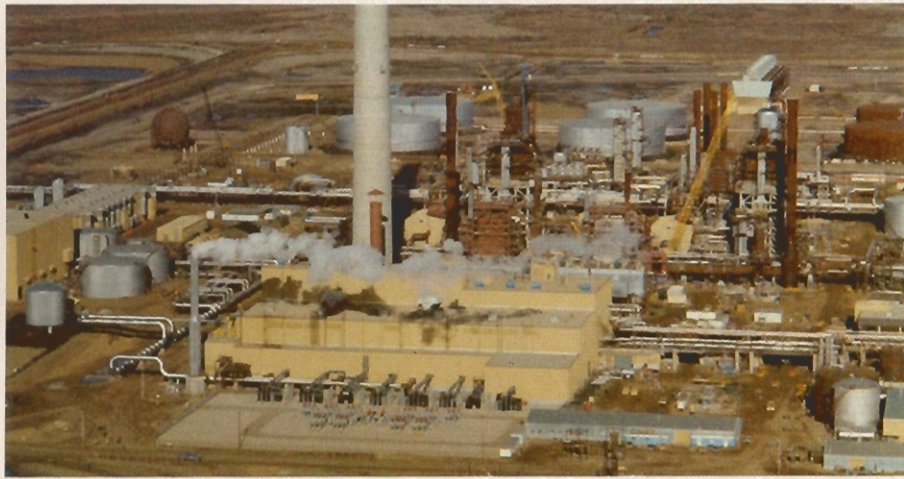
Syncrude Utilities Plant
