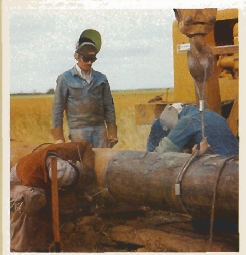
Construction on ethane gathering system
