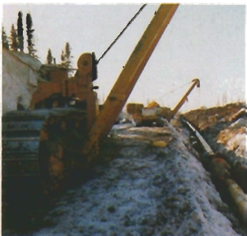
Pipeline crew near the Syncrude site
