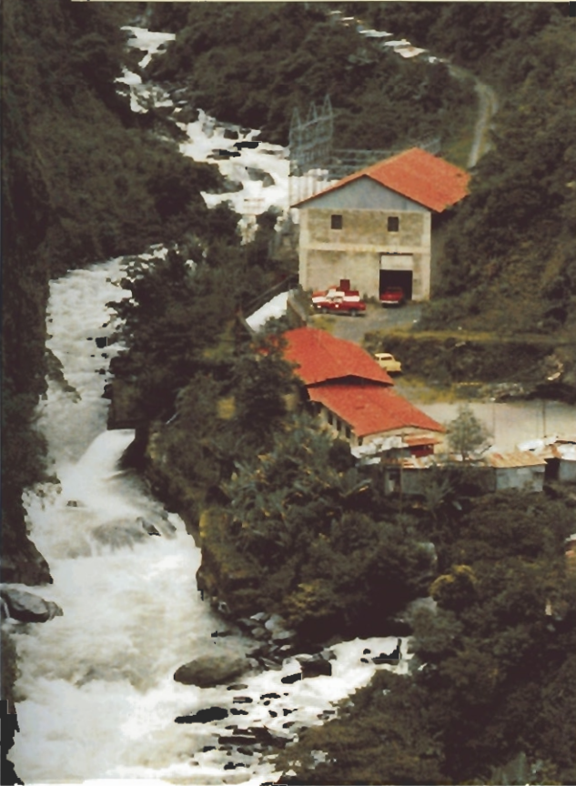
Bolivia Power Company's hydro facilities in the Zongo Valley, near La Paz. AGRA has worked with BPC since 1910
