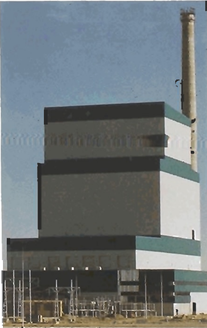
The Shand Power station near Estevan, Saskatchewan is on schedule for completion in 1992. CI Power performed engineering design work on the 300 MW lignite-fired plant in a joint venture for SaskPower.
