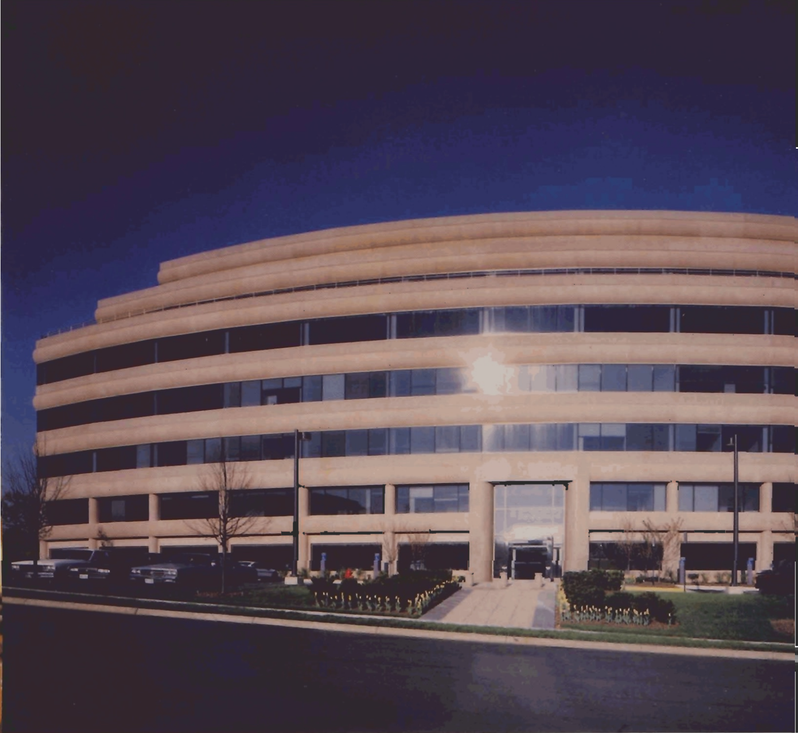
The Williams Plaza in Fairfax, Virginia shows the striking exterior typical of the many U.S. buildings which employ architectural precast concrete panels manufactured by Beer Precast Concrete Limited. Located in a revitalized city center, the office building features bullnose panels with a flamed granite finish.
