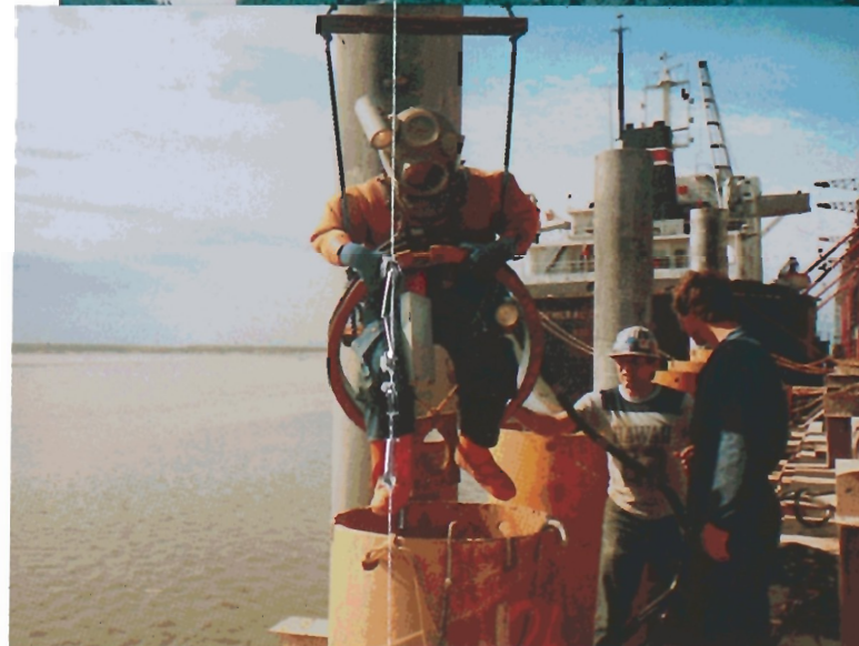
Western Caissons' diver prepares to go down 100 feet in caisson to inspect and cut steel pipe at Churchill's deep sea port on Hudson Bay.
