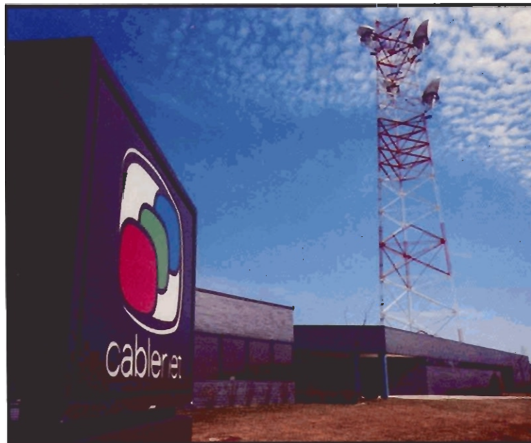
Office and head end for Cablenet Inc. located in Mount Prospect, Illinois just outside of Chicago.
