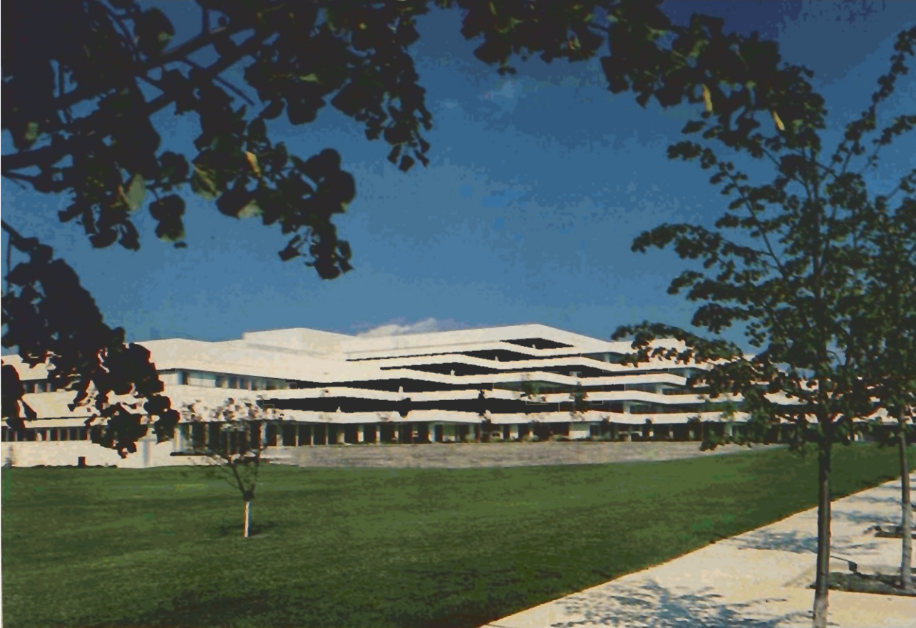
Beer Precast supplied and installed insulated architectural wall panels for the National Revenue Taxation Centre in Sudbury.
