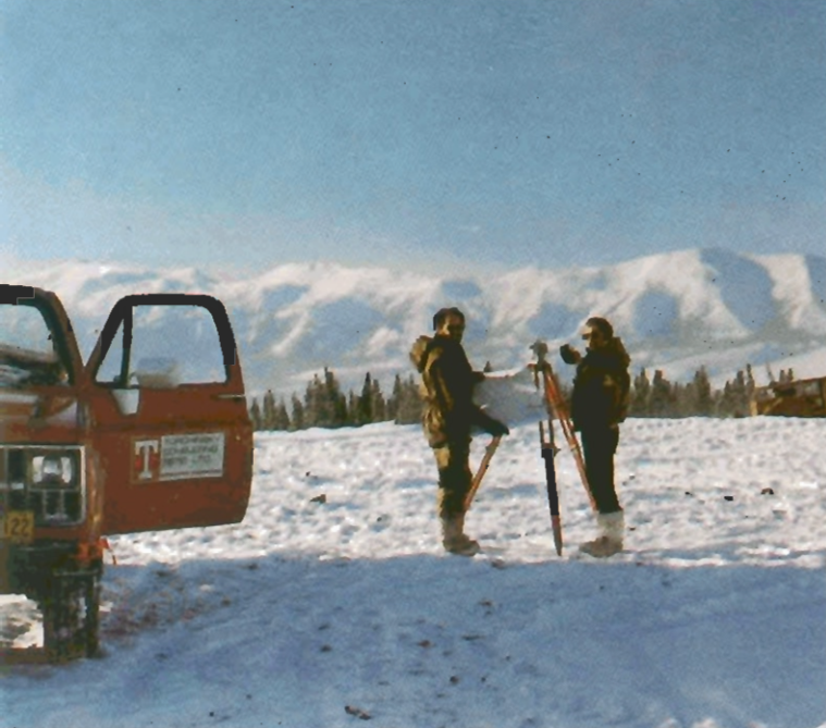
Torchinsky Consulting Party Chief Rick Lisitza and Supervisor Jim Kruse prepare to set survey stakes for Amoco's wellsite development at the Pointed Mountain gas field in the Northwest Territories.
