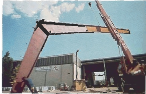
Coast Steel Fabricators produced this rigid frame section.
