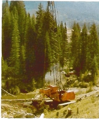
Meredith Drilling installs power line foundations in Colorado. ▶
