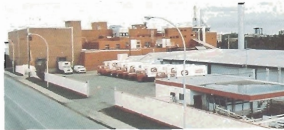
Exterior view of Gainers plant in Edmonton.
