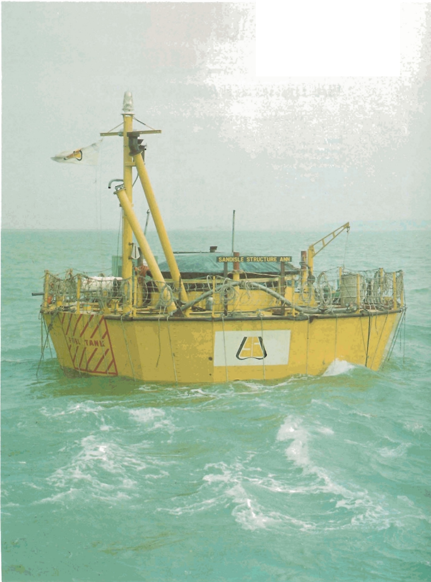
Sandisle Ann is a prototype artificial sand island which was recently successfully constructed in the English Channel five miles offshore in 50 feet of turbulent seas
