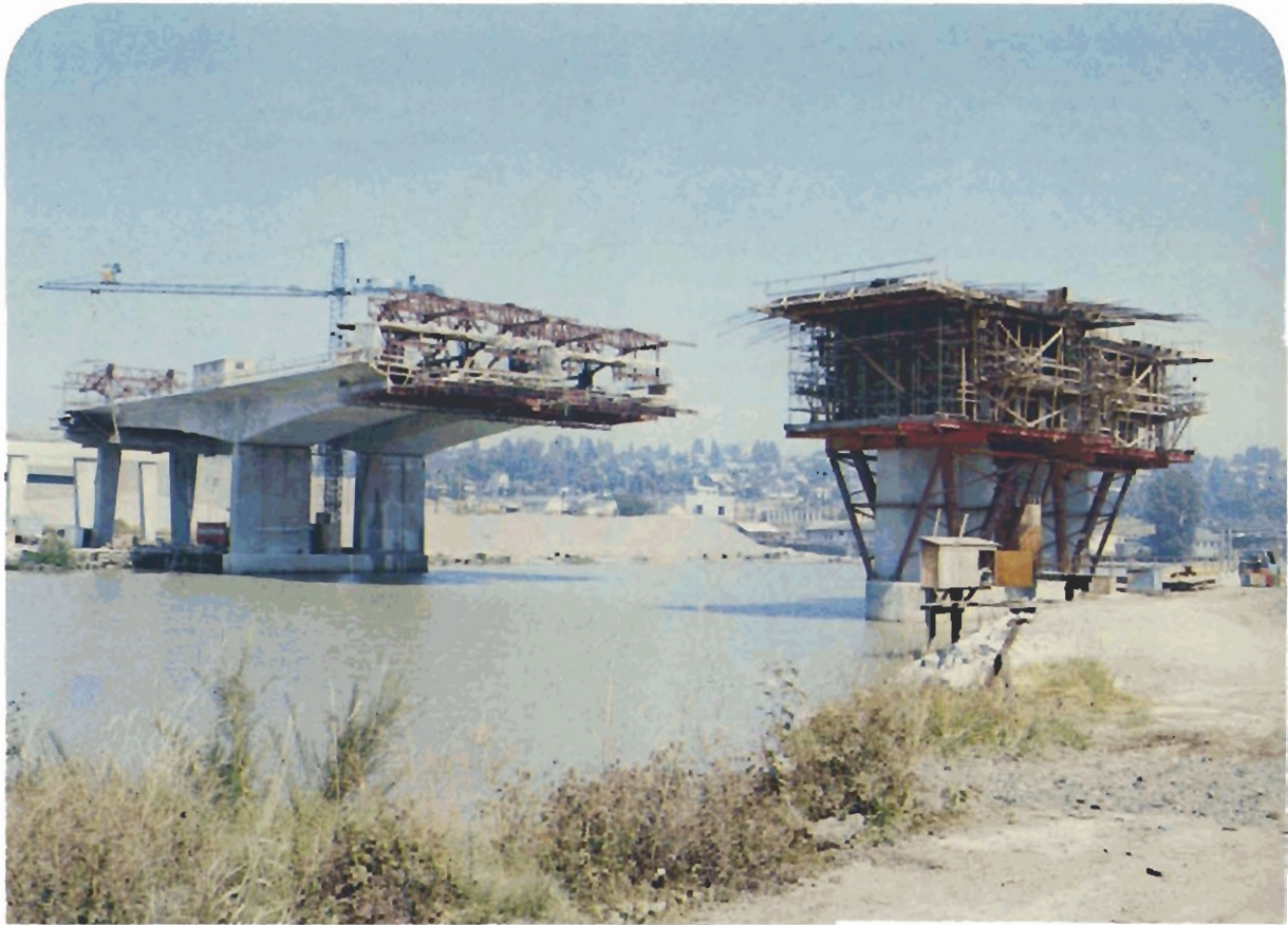
Top — Greenlees Piledriving installed the foundation piles for the approaches of the Knight Street Bridge shown under construction in Vancouver.
