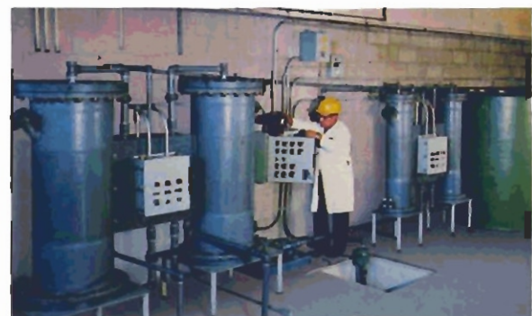
Bottom — One of the field engineers with Cambrian Processes, commissions the pollution abatement facilities designed and built by Cambrian for treating acid pickling wastes at Ontario Malleable Iron Division, ITT Grinnell Company of Canada Ltd. in Oshawa.
