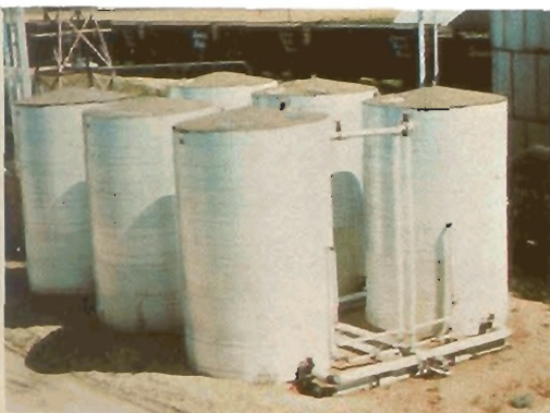
Edible Oil Storage Tanks in Nipawin
