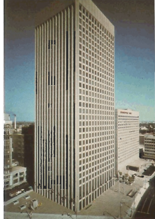
Richardson Tower in Downtown Winnipeg is Supported on Caissons Installed by Western Caissons.
