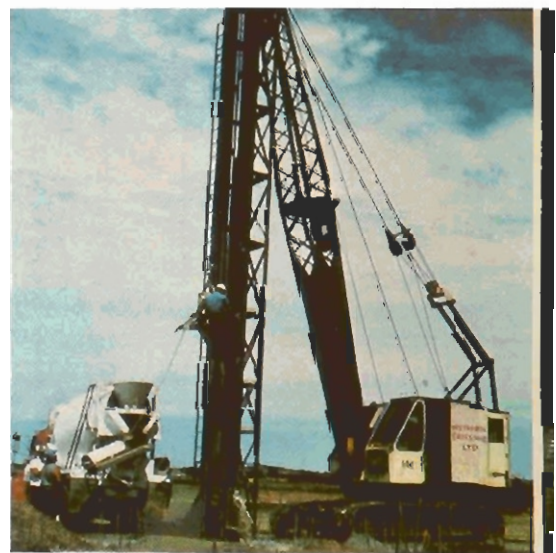
Western Caissons Install Compact-O-Piles in Edmonton
