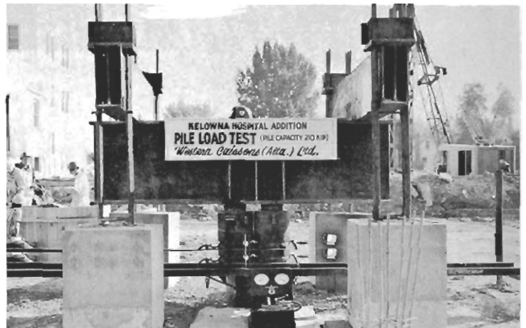
Caisson Load Test
