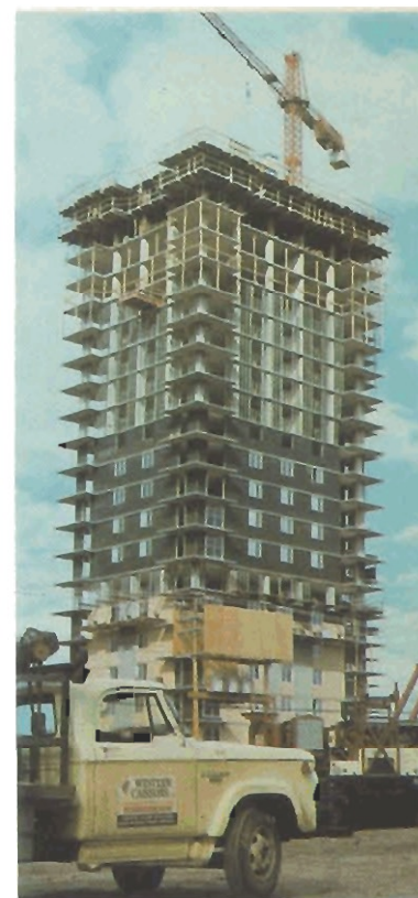
Belled Caissons for Edmonton High-Rise Apartment by Western Caissons
