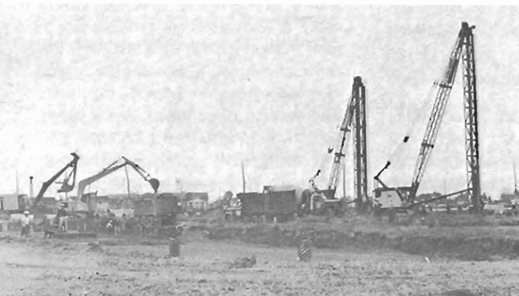
Compact-O-Pile Installation for Ecole Polyvalente Secondaire in Valleyfield, Quebec
