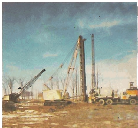
Compact-O-Pile Installation by Western Caissons
