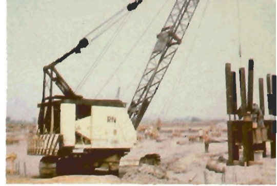
Western Caissons, Driving Pipe Piles for Overpass Structure
