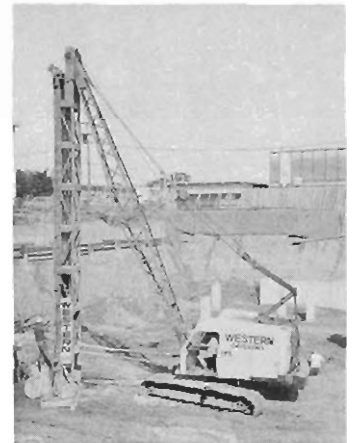
Foundation Piles for 20-Story Apartment in Edmonton
