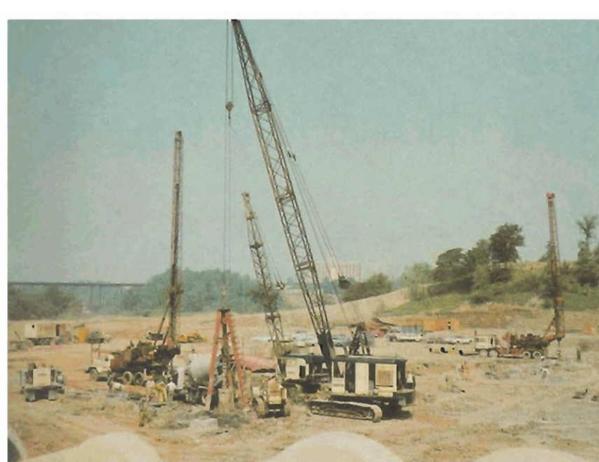
Caissan Installtion for Ontario Science Centre—Toronto's Centennial Project
