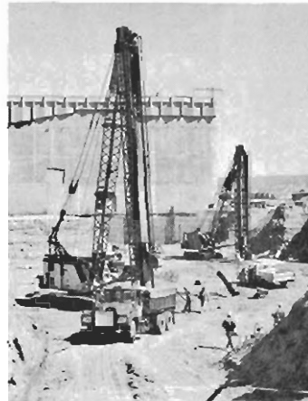
Compacto-Piles for Civil Engineering Building, University of Calgary
