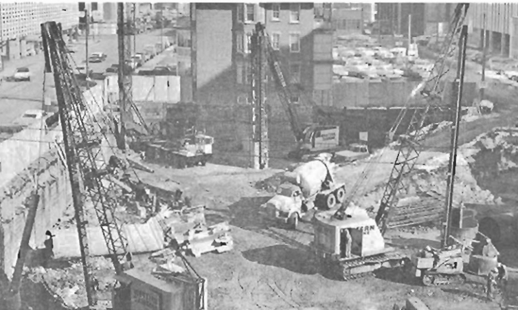
Caisson Installation for Standard Life Building, in Downtown Calgary
