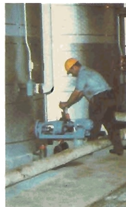
Oil Refinery Storage Tanks
