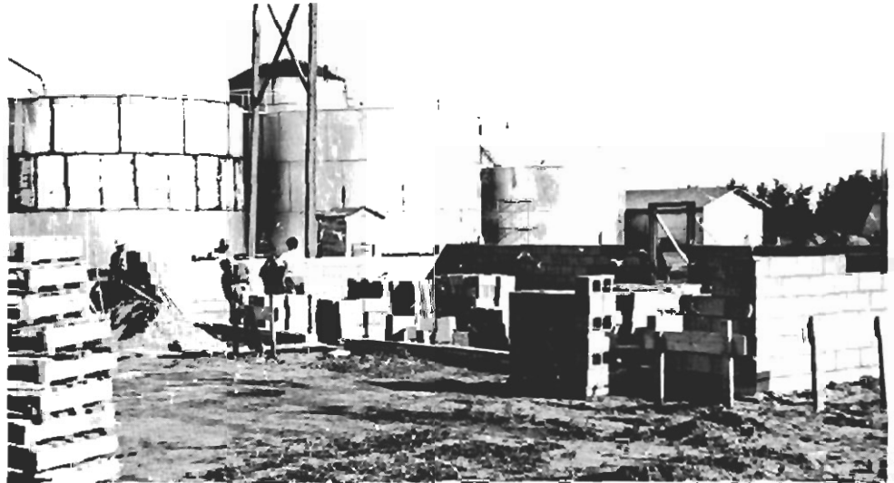
Block laying for new boiler room to service the refinery.
