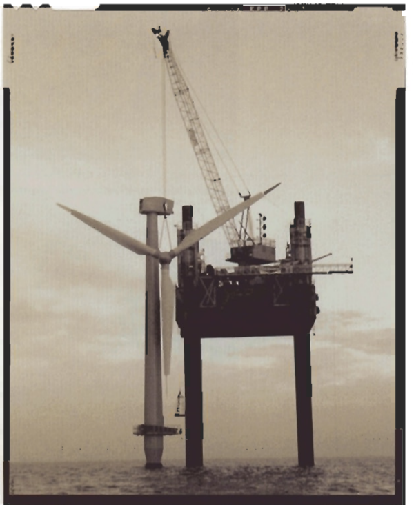
WIND POWER MARINE FOUNDATIONS, BY SEACORE LIMITED IN DENMARK
