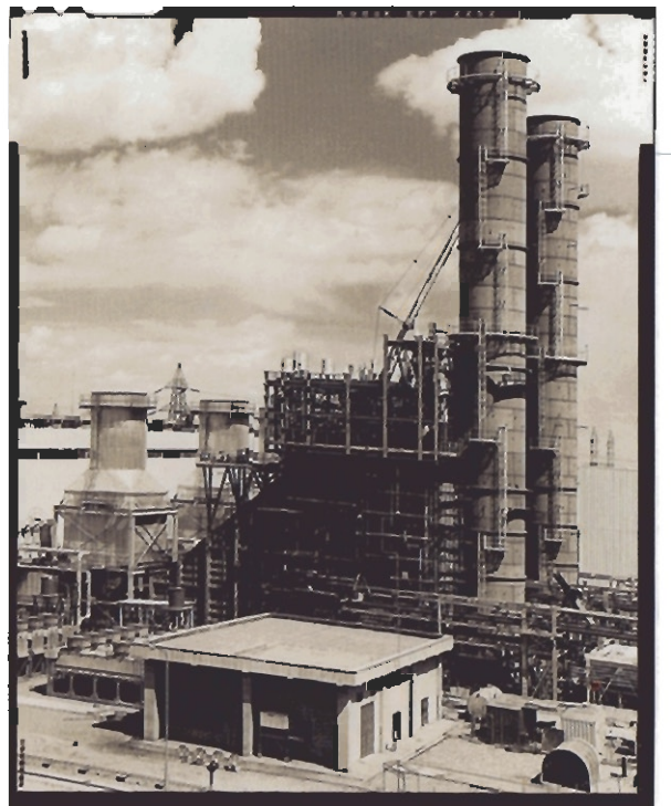
THERMAL POWER PROJECT, MIDDLE EAST
