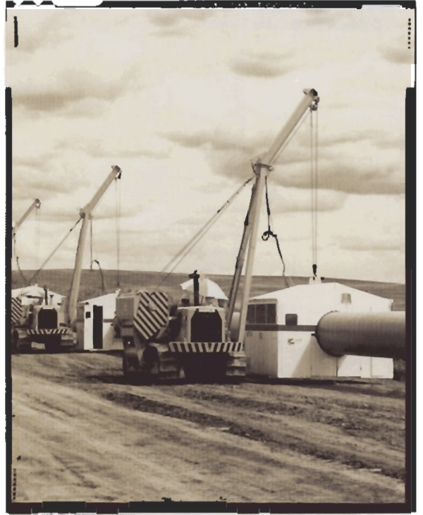
PIPELINE CONSTRUCTION, ALBERTA
