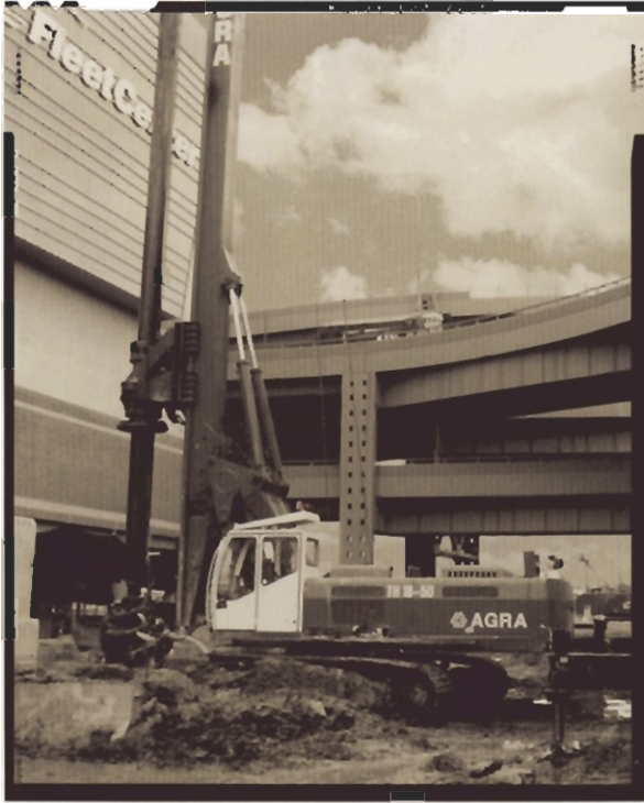
FOUNDATION CONSTRUCTION, CENTRAL ARTERY PROJECT, BOSTON
