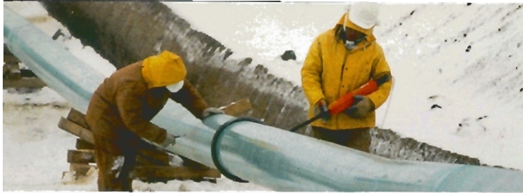
Pipeline construction work— United States
